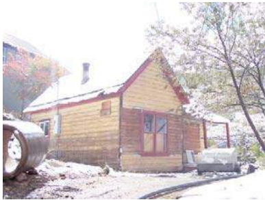
68 PROSPECT STREET Landmark Site
