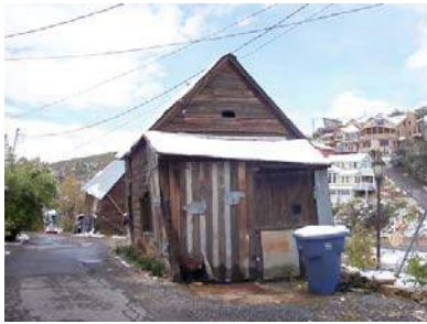
152 SANDRIDGE AVENUE Accessory Building
