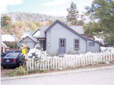
39 SEVENTH STREET Landmark Site
