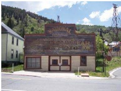
703 PARK AVENUE GARAGE (Pre-rehab) Landmark Site
