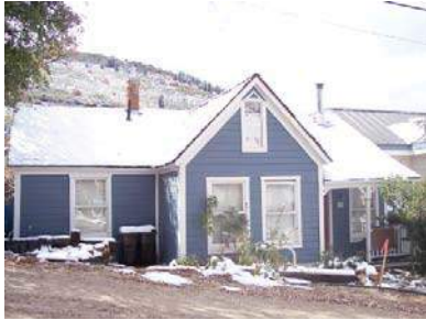
36 PROSPECT STREET Landmark Site
