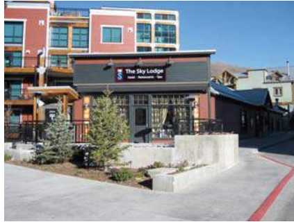
201 HEBER AVENUE Significant Site
