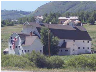
3000 Highway 224 (Total of six structures) Landmark Site
