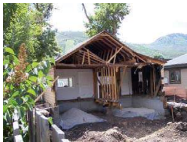
1326 PARK AVENUE (rear-during construction)
