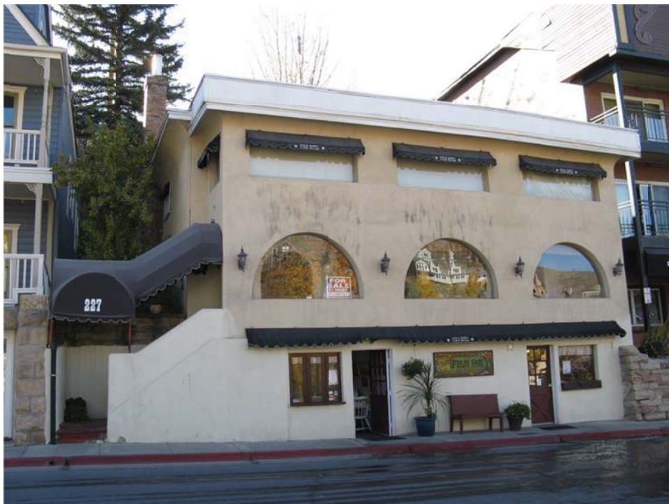
227 Main Street. Southeast oblique. October 2013.
