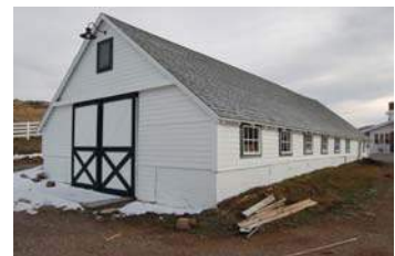
2414 MONITOR DRIVE Accessory Building
