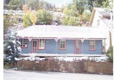
118 DALY AVENUE (pre-partial Reconstruction) Significant Site
