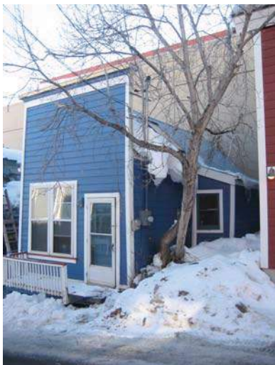
120 FOURTH STREET Significant Site
