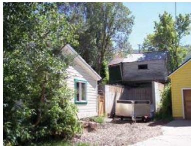
1439 WOODSIDE AVENUE Accessory structure
