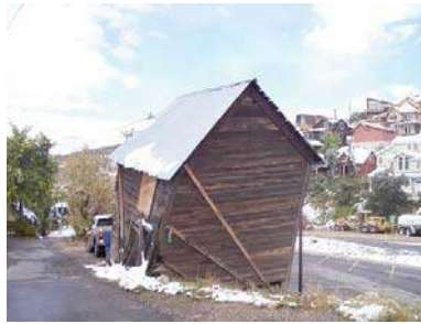
156 SANDRIDGE AVENUE Accessory Building
