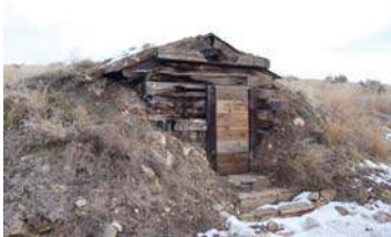
2414 MONITOR DRIVE Structure
