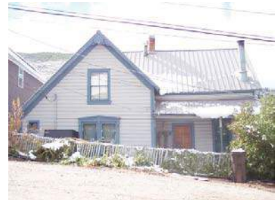
22 PROSPECT STREET Landmark Site
