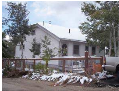
101 PROSPECT STREET Landmark Site
