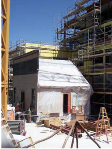
199 HEBER AVENUE Significant Site
