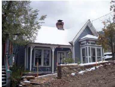
59 PROSPECT STREET Landmark Site
