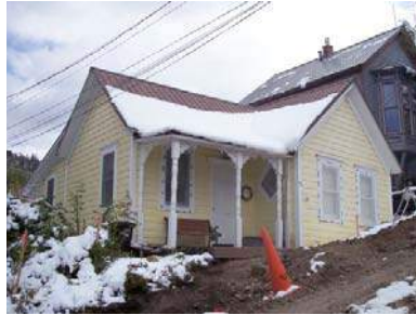
51 PROSPECT STREET Landmark Site
