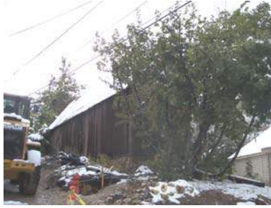
9 HILLSIDE AVENUE (pre-reconstruction)
