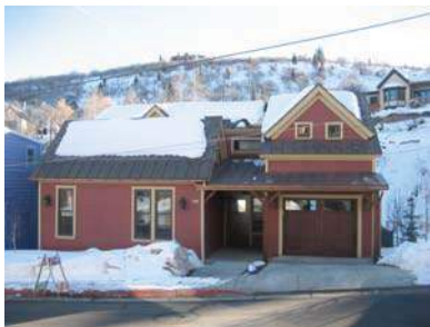
148 MAIN STREET (aka 130 Grant Avenue) Significant Site
