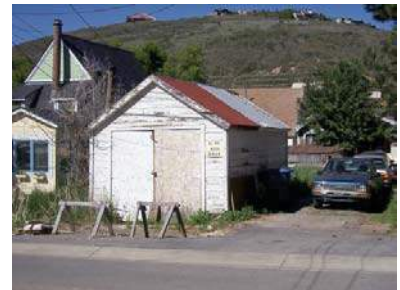
1043 PARK AVENUE Accessory Building
