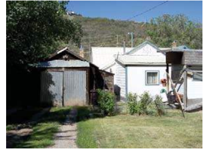
1141 PARK AVENUE Accessory Building
