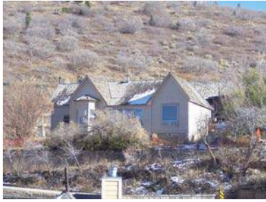
9 HILLSIDE AVENUE (pre-reconstruction) Significant Site
