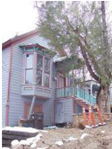
57 PROSPECT STREET Landmark Site
