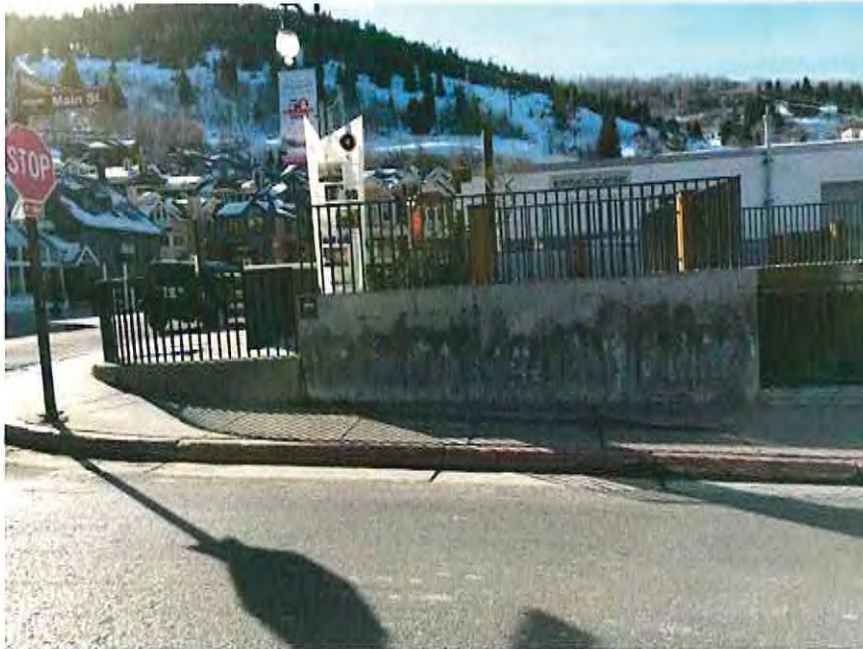
38 Main Street - Rectangular Black Steel Street-side Railing
