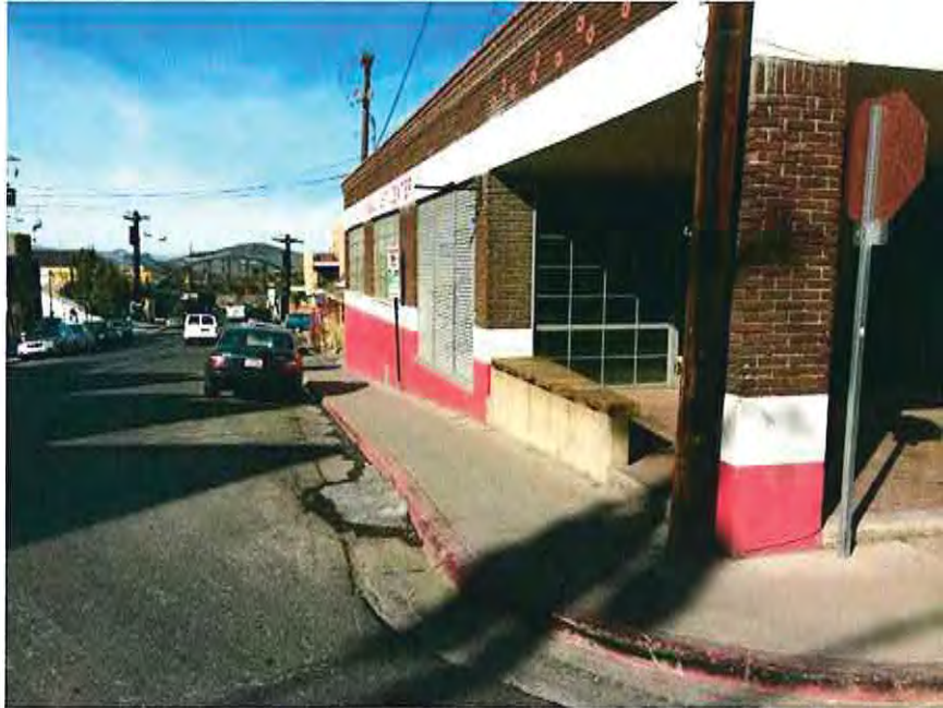
1 Corner Heber Ave & Park Ave - Looking North
