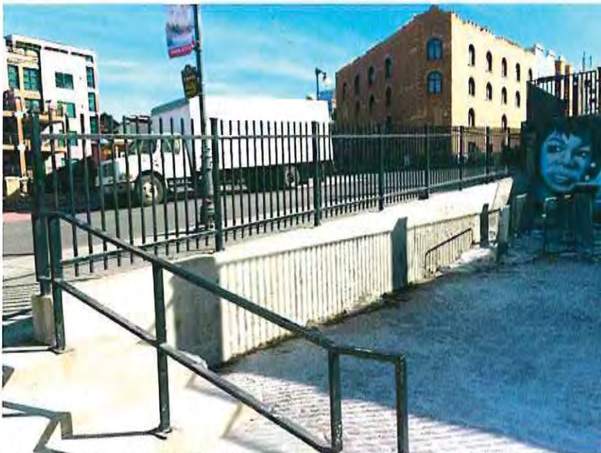
31 Main St - Black Steel Fence above Retaining Wall Cont.
