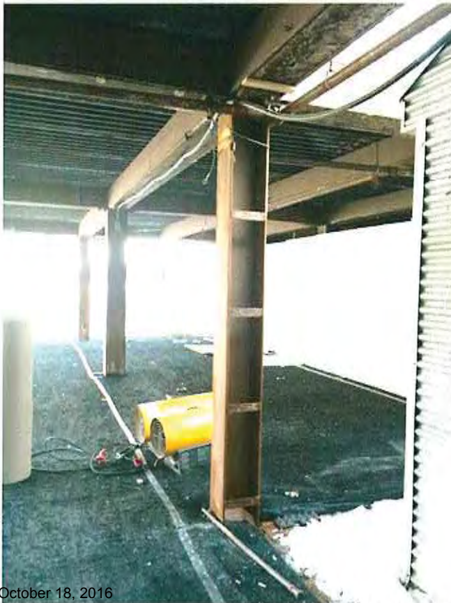
79 Patio Level - Exterior I Column, & Beam W/ Metal Decking
