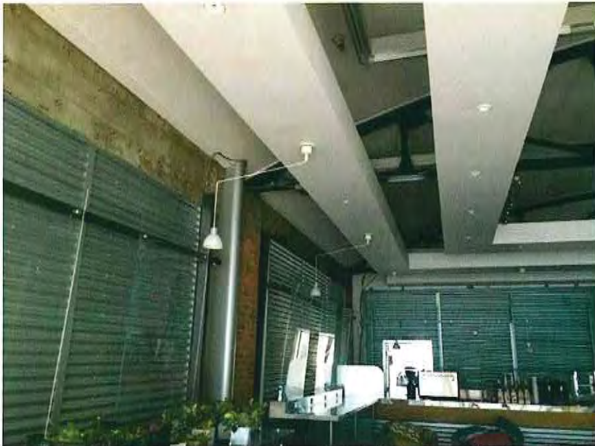
81 Level 1 - Bow Truss Roof on Brick/Concrete Columns
