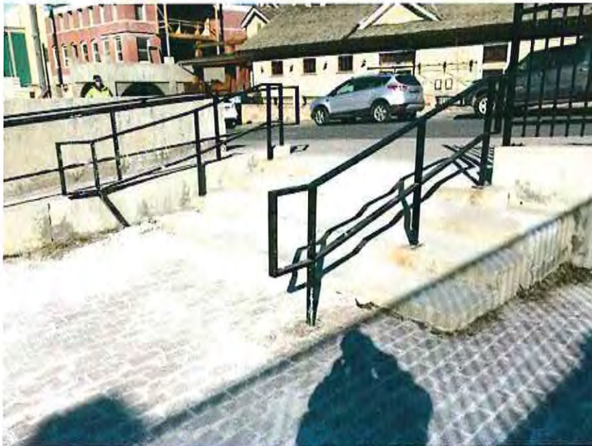
37 Patio - Rectangular Black Steel Stair Railing
