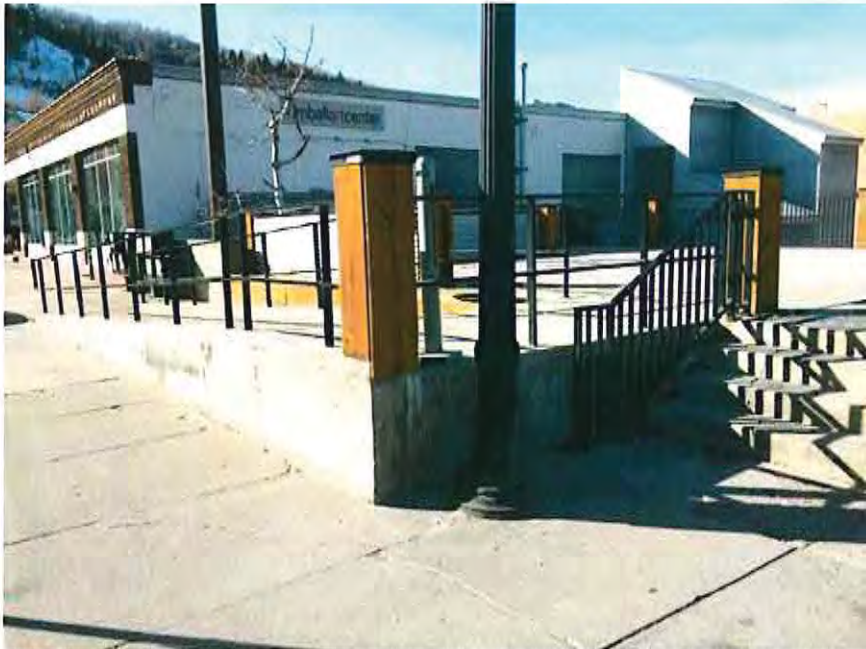
35 Deck to Heber Ave Sidewalk - Rectangular Black Steel Stair and Ramp Railing with Stained Timber Posts
