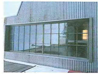
Storefront Detail - East Wall
