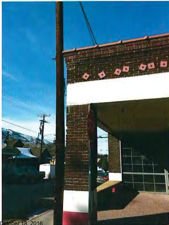
83 Level 1 - Exterior Concrete/Brick Column on Slab on Grade
