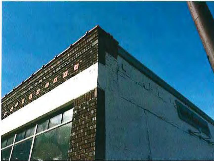
42 Exterior Brick Cornice and Metal Flashing
