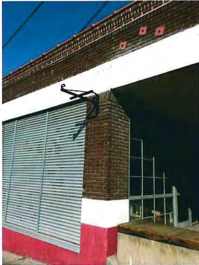
82 Level 1 - Exterior Concrete/Brick Column on Slab on Grade
