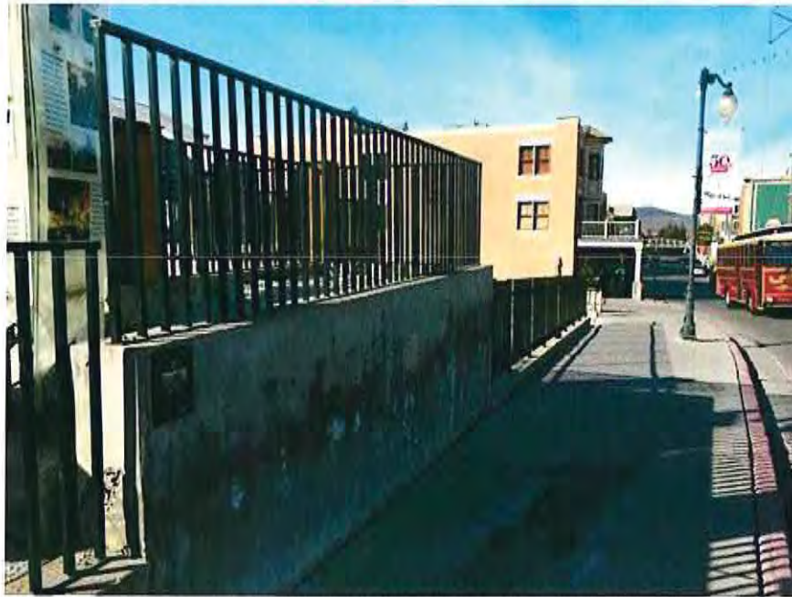
4 Corner Main St & Heber Ave - Looking North
