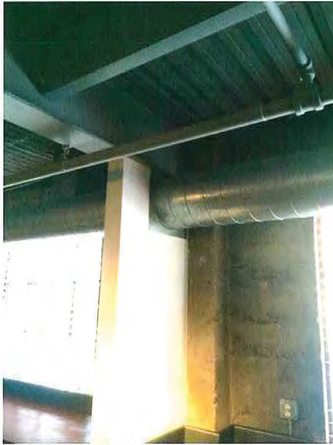
78 Patio Level - Interior Beam on Concrete Column W/ Patched Metal Decking
