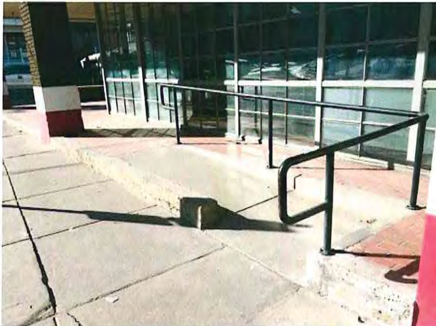
26 Heber Ave to Main Entrance - Concrete Ramp
