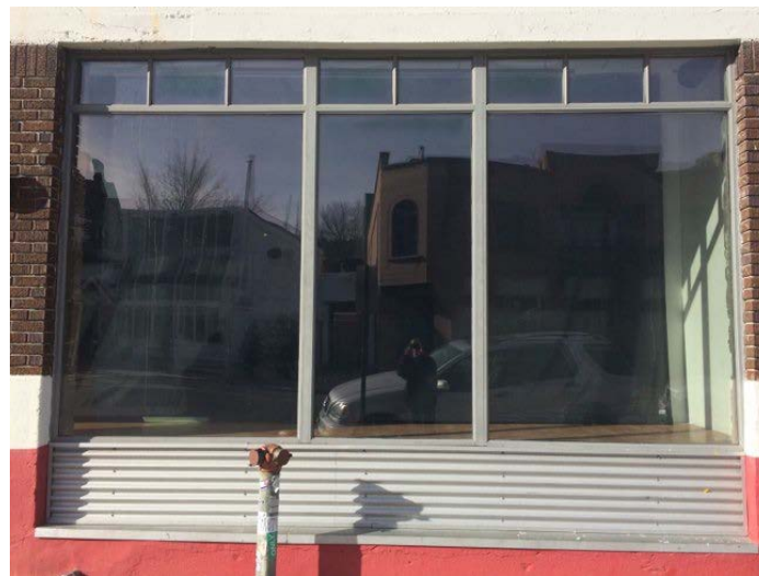
Figure 15. Typical replacement window and corrugated metal bulkhead along Heber Avenue.
