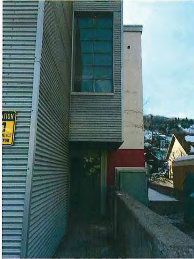
66 Stairwell & Elevator Shaft Addition - North Face
