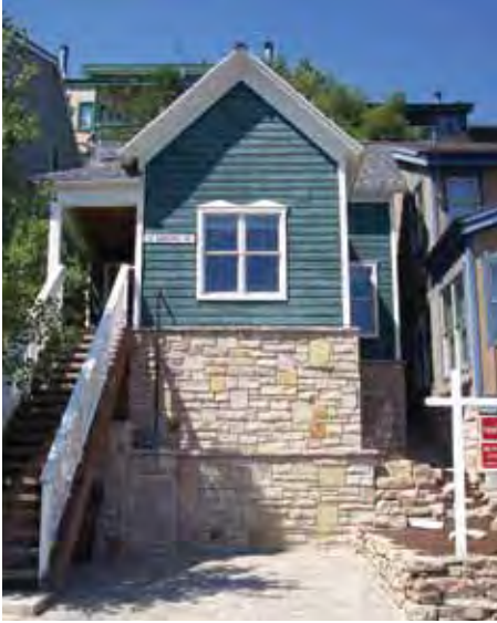
Landscaping and site grading, particularly in the front yard setback, are important elements in defining the character of the street. Unlike the example above, original grading in the front yard setback and compatible landscaping should be maintained.
