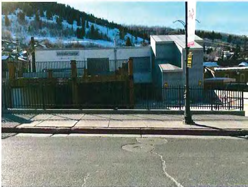
30 Main St - Black Steel Fence above Retaining Wall
