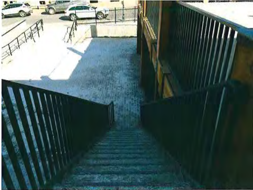
34 Deck to Patio - Rectangular Black Steel Stair Railing
