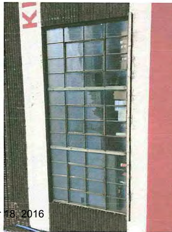
Storefront Detail W/ Operable Glazing - East Facade
