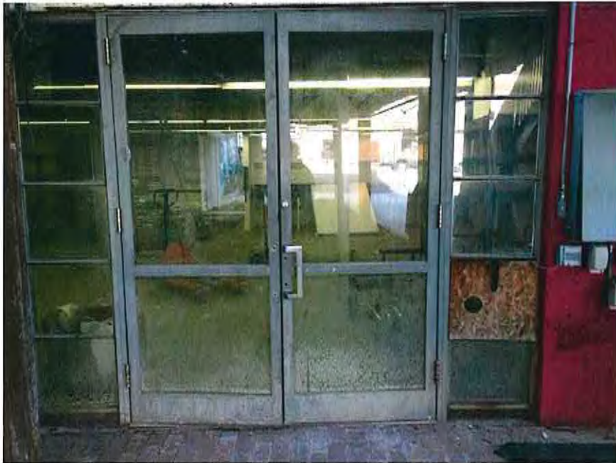
102 Patio Level - #3 Entry Storefront
