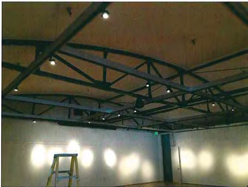
43 Bow-truss Roof Shape
