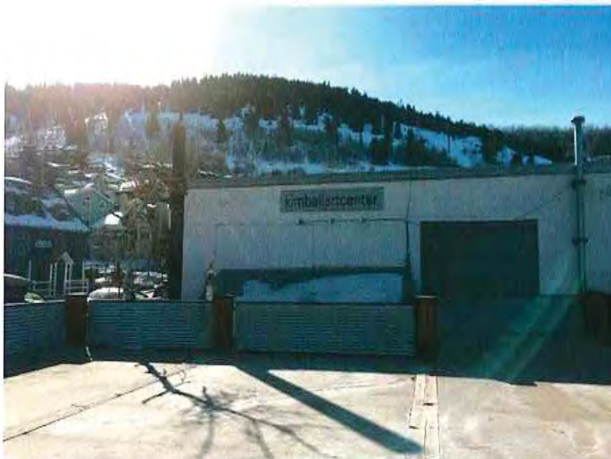
33 Deck - Corrugated Aluminum Railing with Stained Timber Posts
