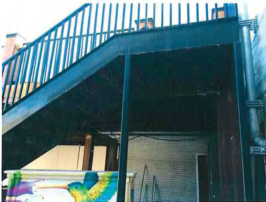
67 Kiln Room & Stair Shaft Addition
