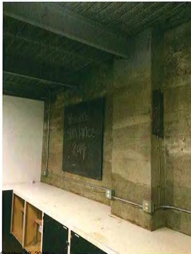
Patio Level - Interior Joists on Concrete Column W/ Original Metal Decking
