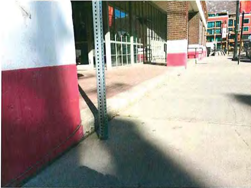
25 Heber Ave to Main Entrance - Concrete Step with Brick Pavers
