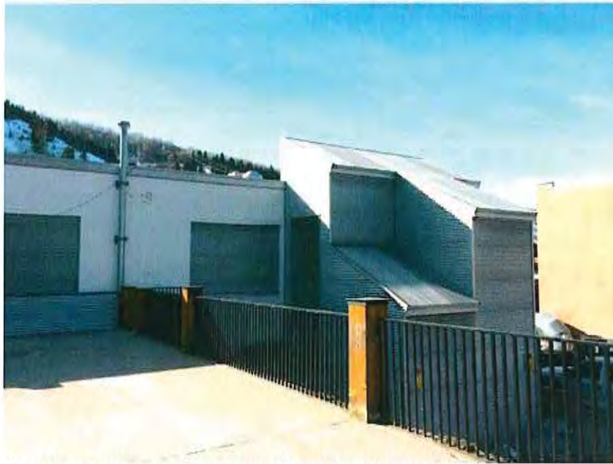
32 Deck - Rectangular Black Steel Railing with Stained Timber Posts
