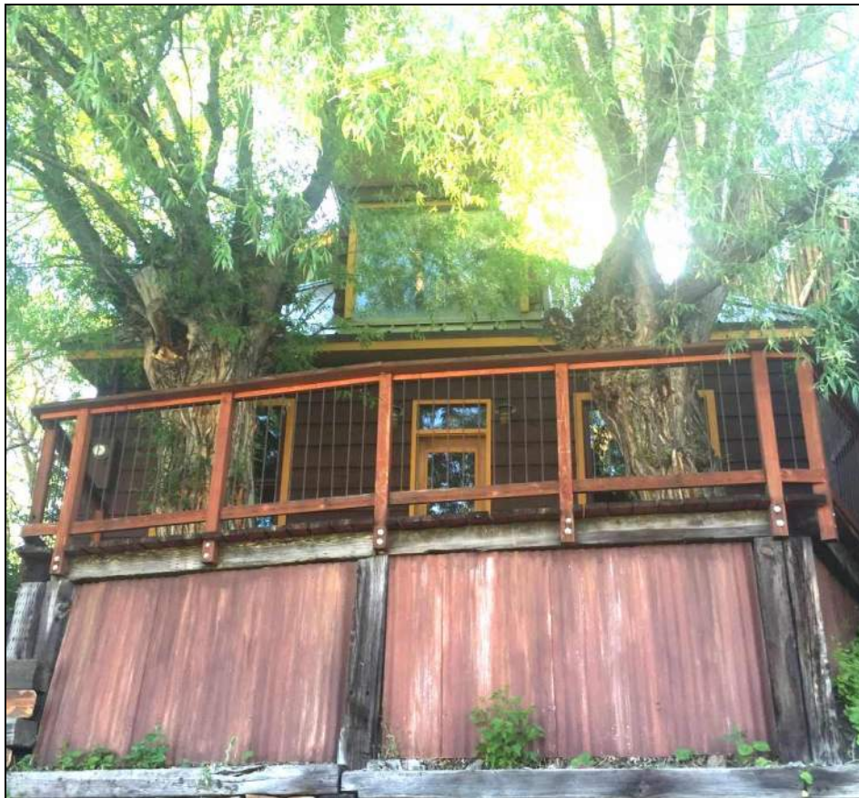
416 Ontario Avenue. West Elevation. June 2016.
