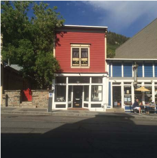
The new building at 525 Main Street (Main Street Deli) maintains the stepping effect, rhythm and pattern of storefront openings, and cornice of the storefront with its historic neighbor at 523 Main Street.
