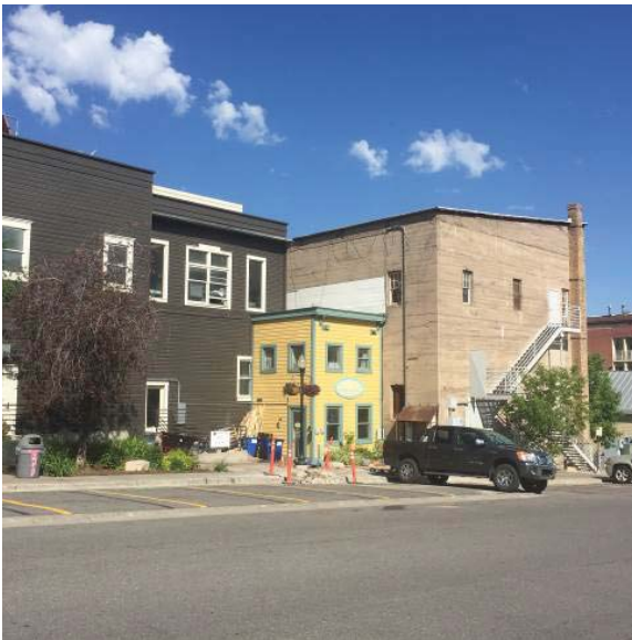
This stairway is installed on the outside of the historic Elks Lodge (550 Main Street) on the Sweede Alley Façade.
