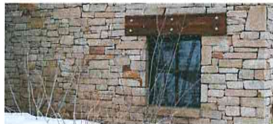
Window is a feature element within this wall plane
