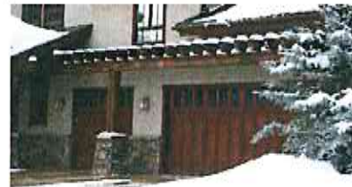
Not this - Garage doors for three cars occur on the same wall plane
