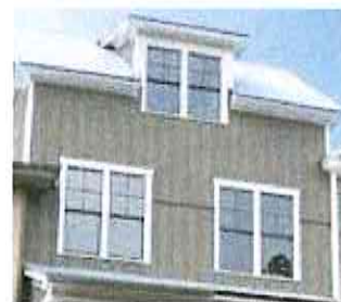
Shutters not prominent in Park Homes
