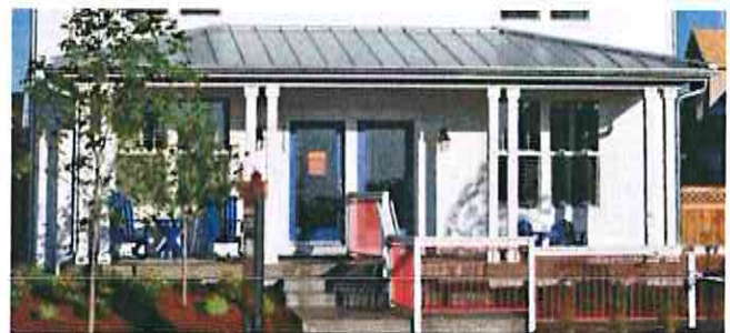
Properly detailed porch elements
