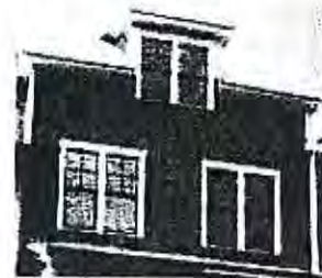
Shutters not prominent in Park Homes
