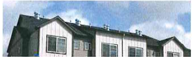
Mechanical vents reflect architectural style
