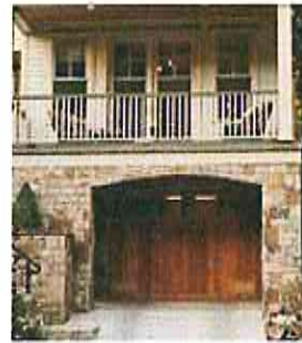
Patio over garage lessens its visual impact
