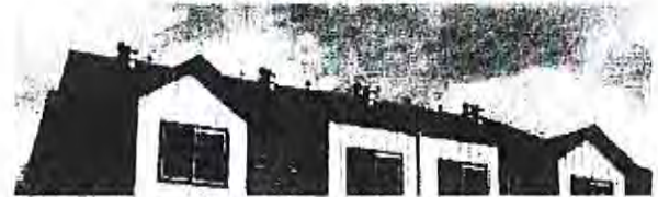
Mechanical vents reflect architectural style
