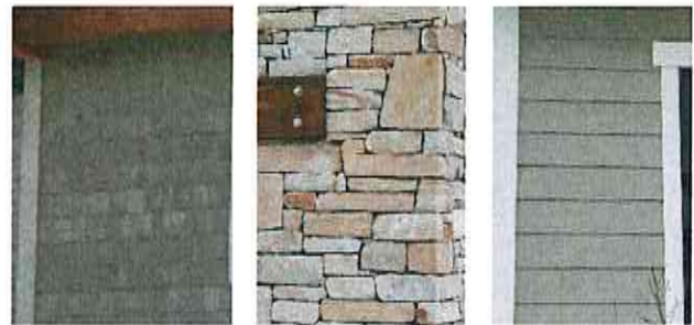
Varied wall materials provide interest and distinction to wall planes
