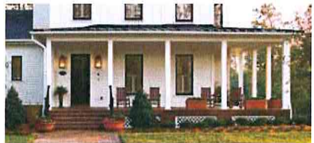
Porch raised above finished grade
