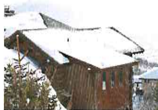
Simple roof forms
