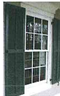
Shutters sized to match openings
