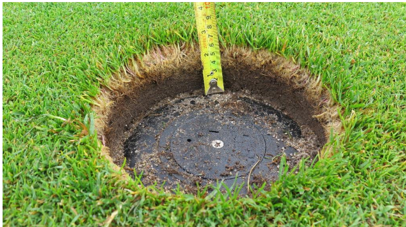
Example of a full-circle sprinkler near a green. The maintenance staff is doing an excellent job at keeping these trimmed and edged, which reduces the potential for water to hit adjacent grass blades that can lower distribution uniformity (DU). However, the greenside sprinklers are low and require leveling.
