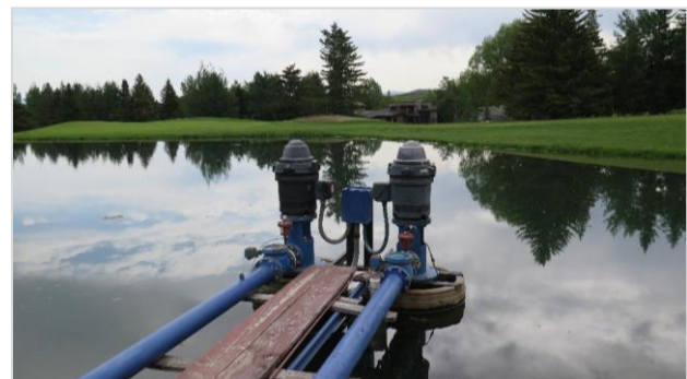
(L) The pump station was installed in 1987 and adjusts water flow and pressure for the irrigation system. (R) The 75-hp pumps are located out over the water and susceptible to deterioration by sun and various other weathering elements.
