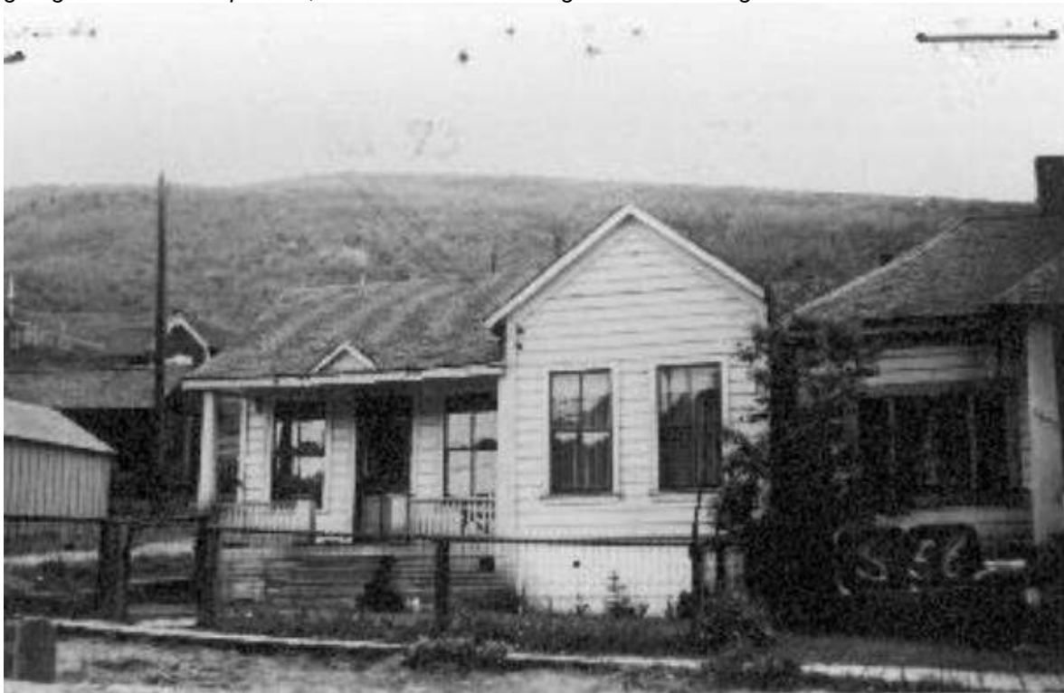
Figure 3: 1103 Woodside Avenue ca. 1940 tax photograph. Visible in this photograph is the single-car garage with its white-painted, board and batten siding and wood-shingled roof.
