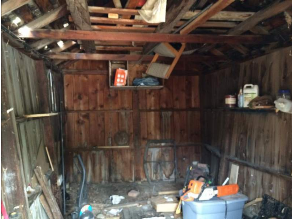
Figure 5. General view of garage interior, facing west.
