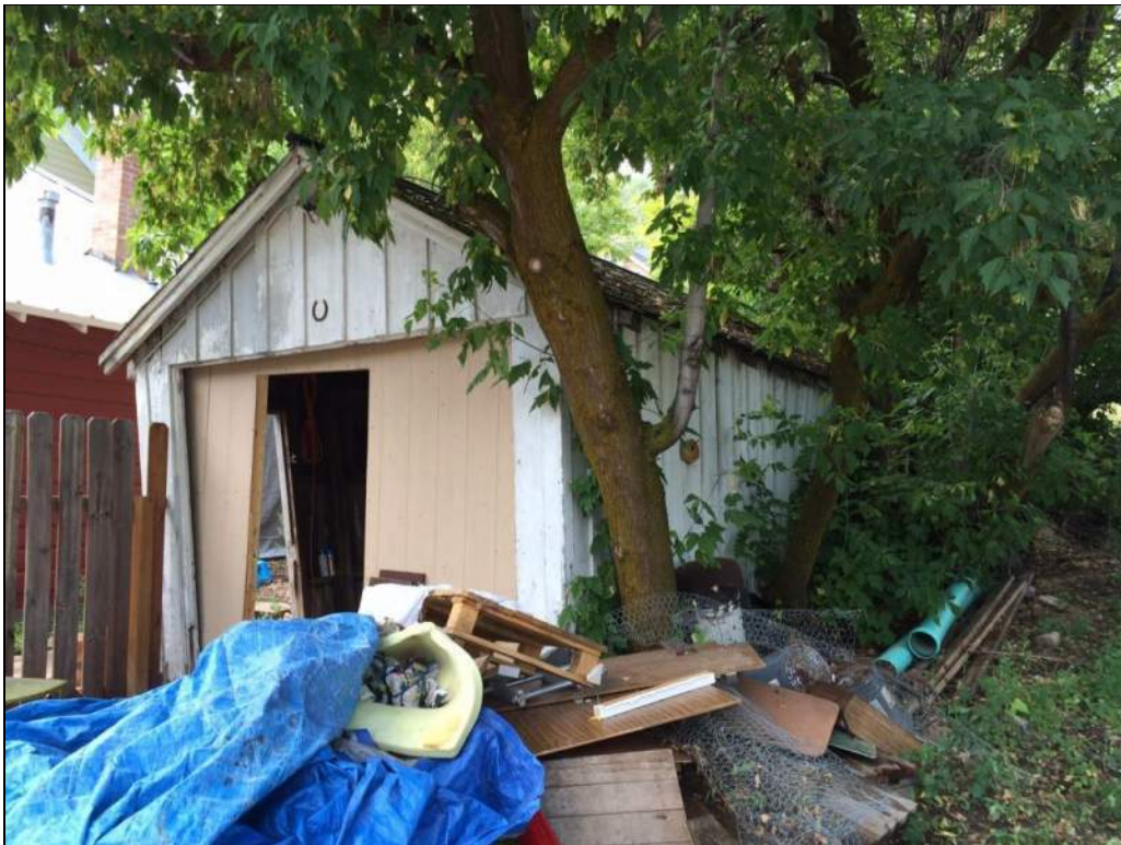
Figure 4. General view of garage, facing southwest.
