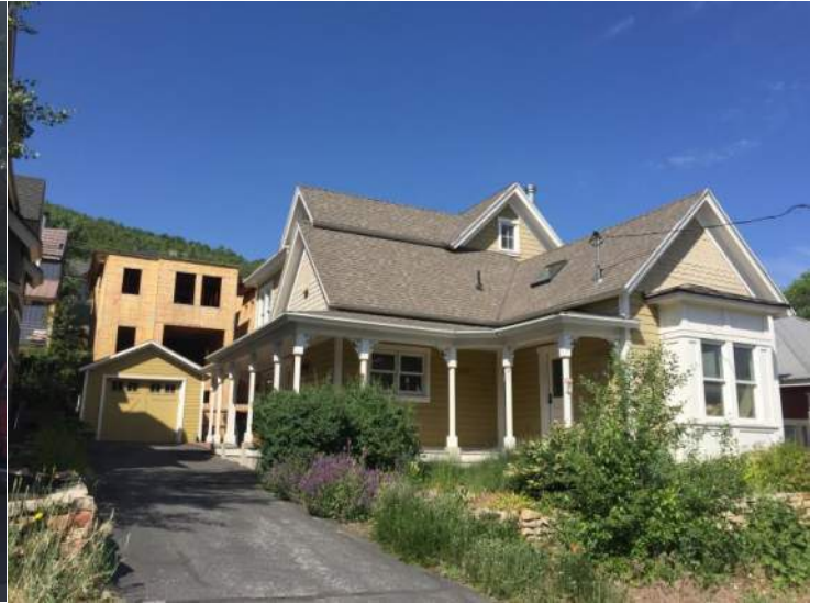
1053 Woodside Avenue located just south of 1057 Woodside Avenue. Note the garage located in the rear yard, yard space, separation between structures. Camera facing northwest.
