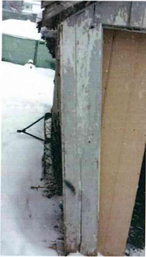
Southeast corner of shed
