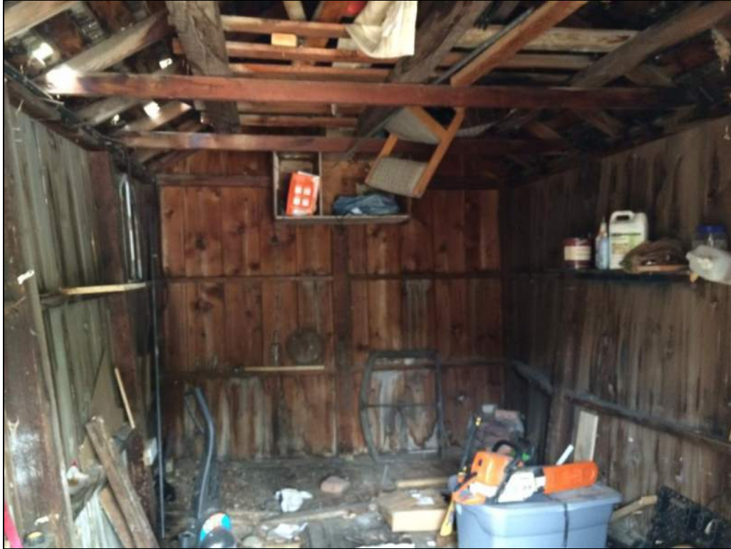
Figure 5. General view of garage interior, facing west.
