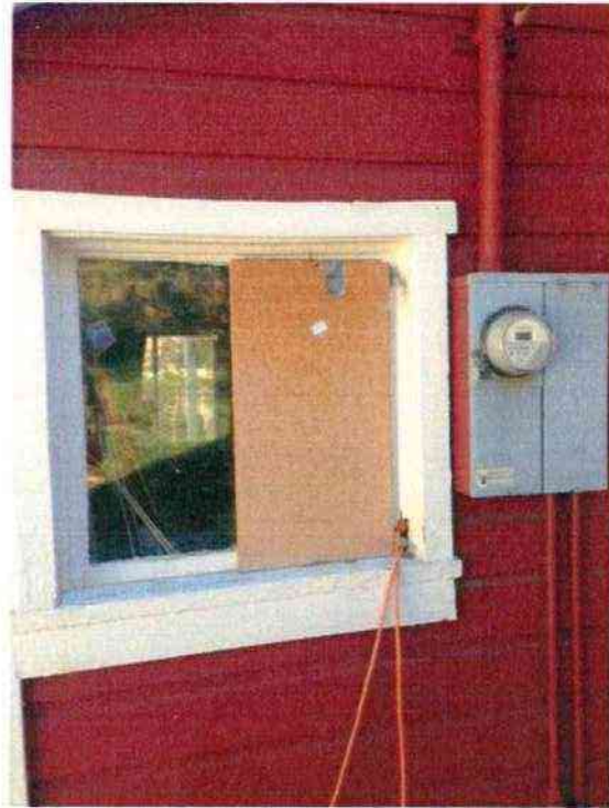
Window #2- Condition- Original/poor
