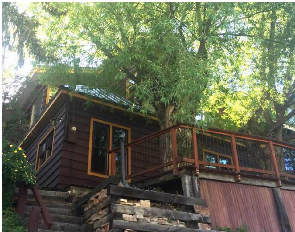
416 Ontario Avenue. Southwest Oblique. June 2016.
