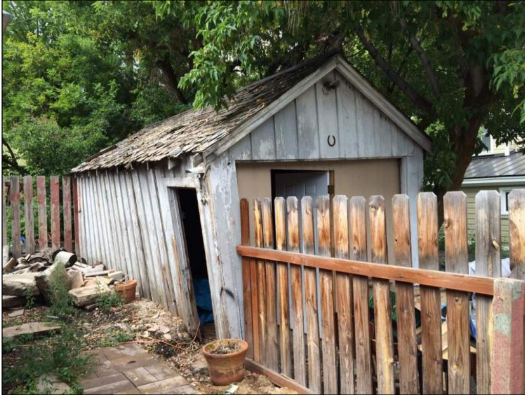
Figure 3. General view of garage, facing northwest.
