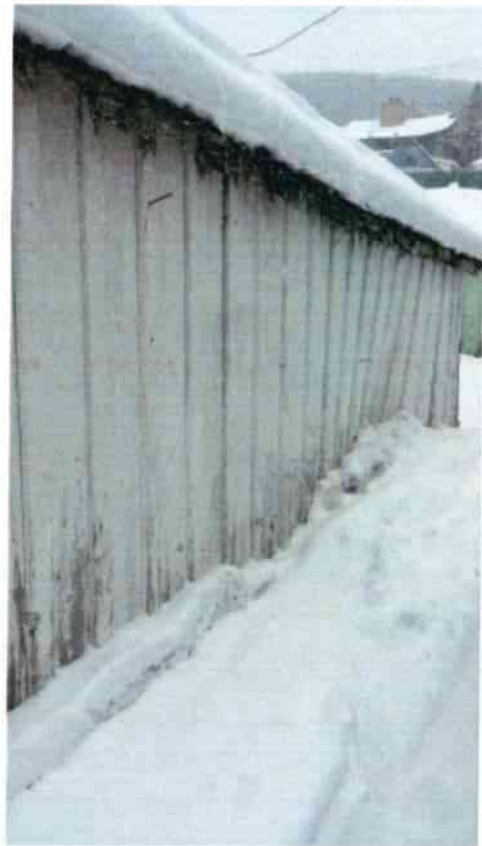
North wall of shed
