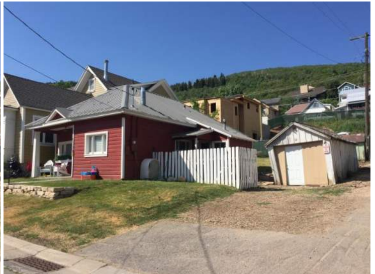
1057 Woodside Avenue (centered). Note the relationship between the single-family dwelling and its outbuilding(s). Camera facing southwest.
