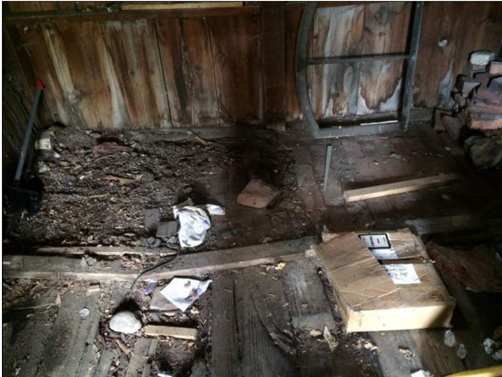
Figure 6. Garage floor, showing brickwork at west end and wood planks covering remainder of floor, facing west.
