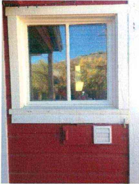
Window #1- condition- Original, poor
