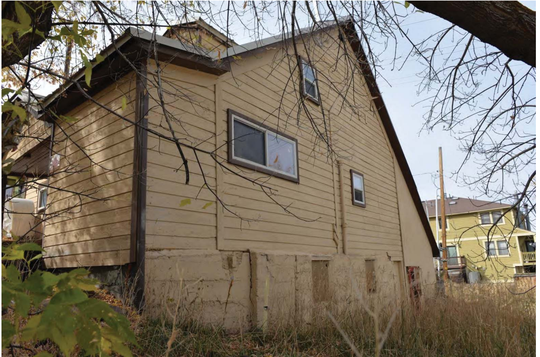
844 Empire Avenue looking northwesterly
