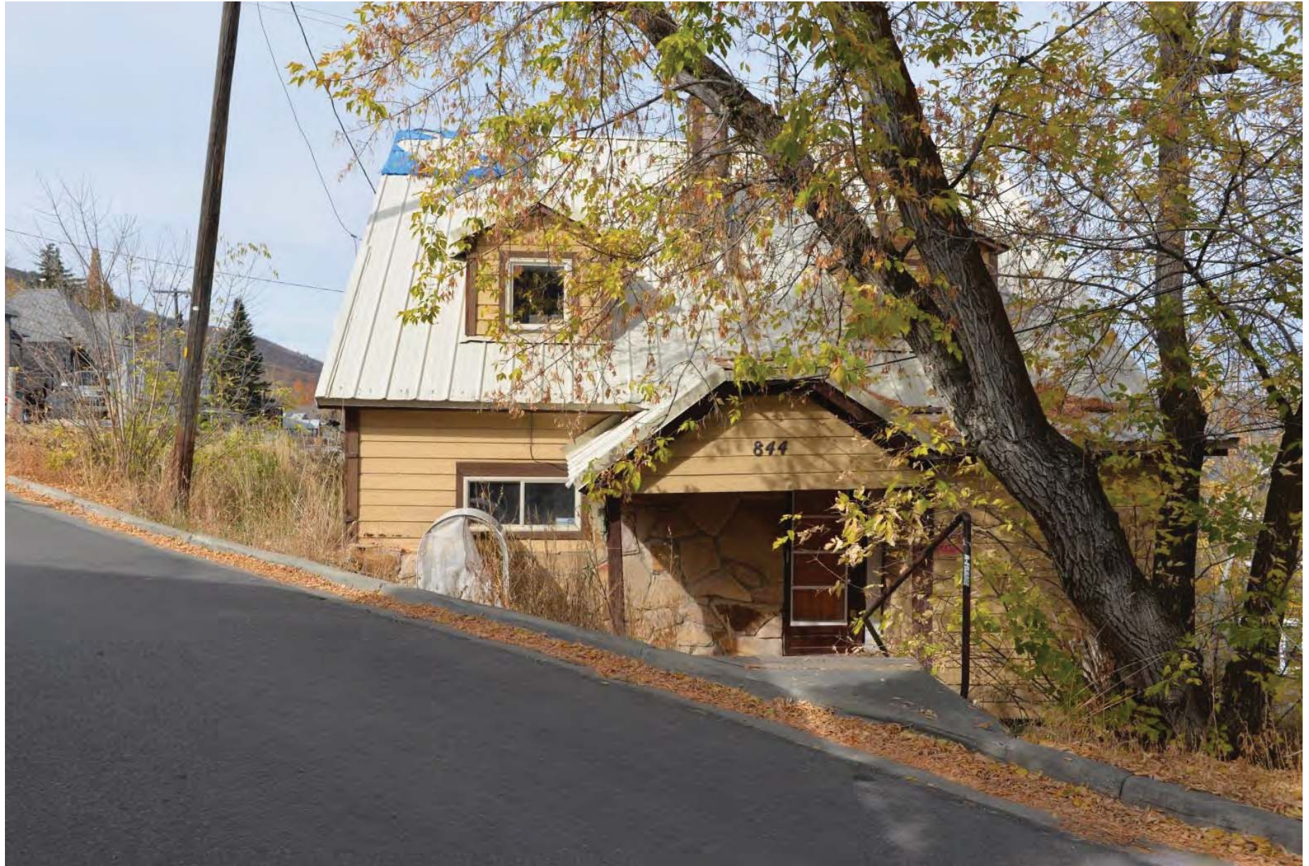
844 Empire Avenue looking northerly
