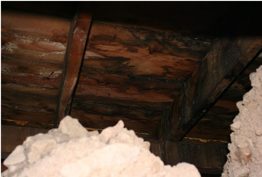
Photo of existing roof structure above the house.
