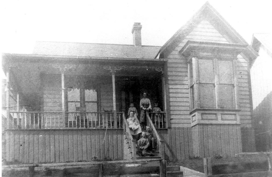
This photograph, taken prior to 1927 shows the original porch, porch's architectural ornamentation, box bay, and original chimney.
