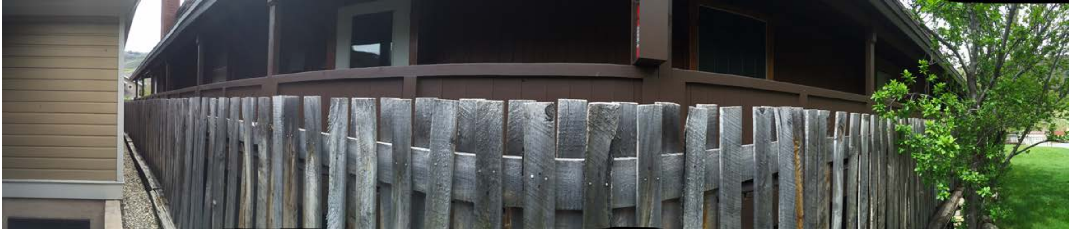
North Side Looking South
