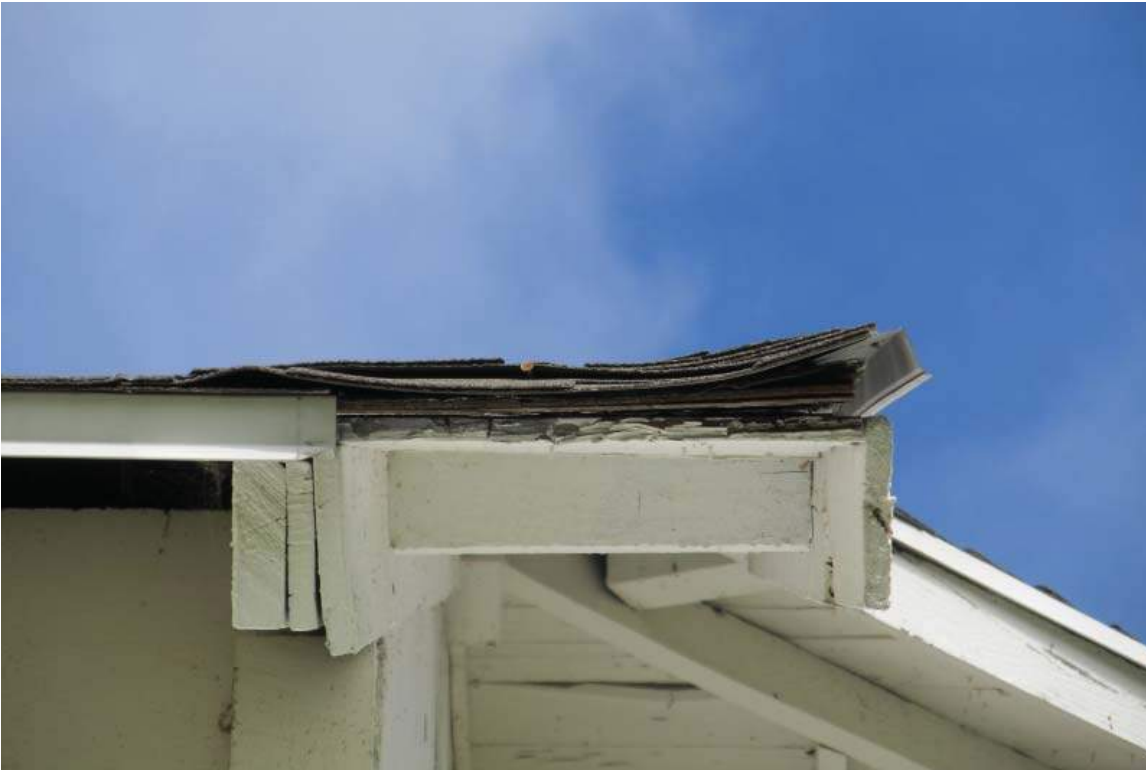
Photo #007: Roof Detail
