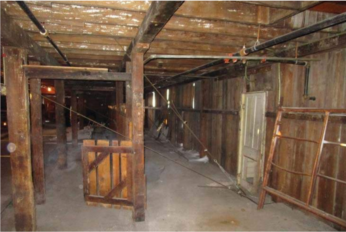
Photo #003: Lower Level Structure
