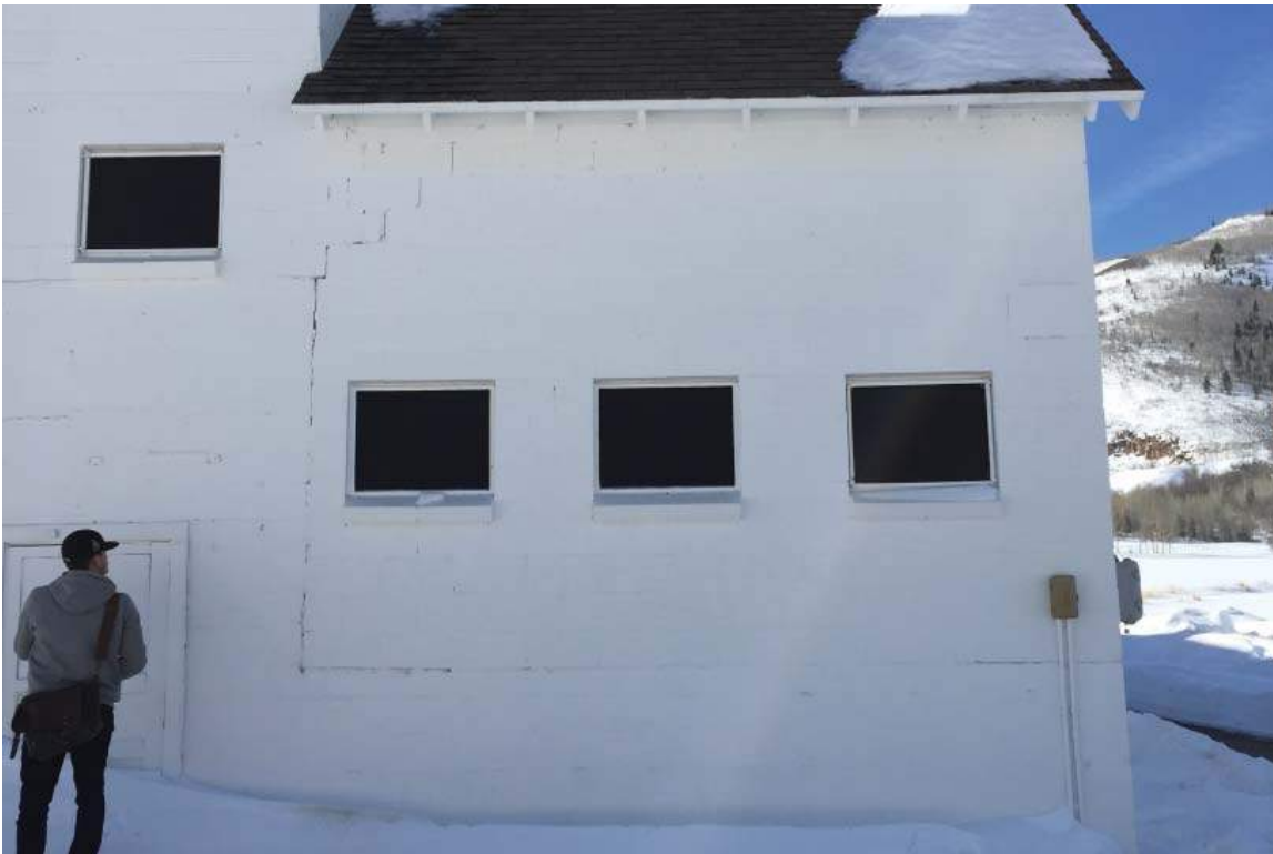
Photo #024: Northwest Addition North Wall
