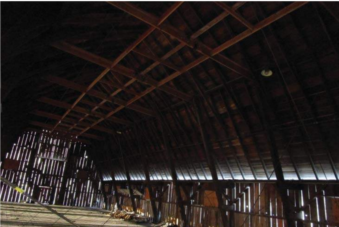
Photo #004: Upper Level Structure
