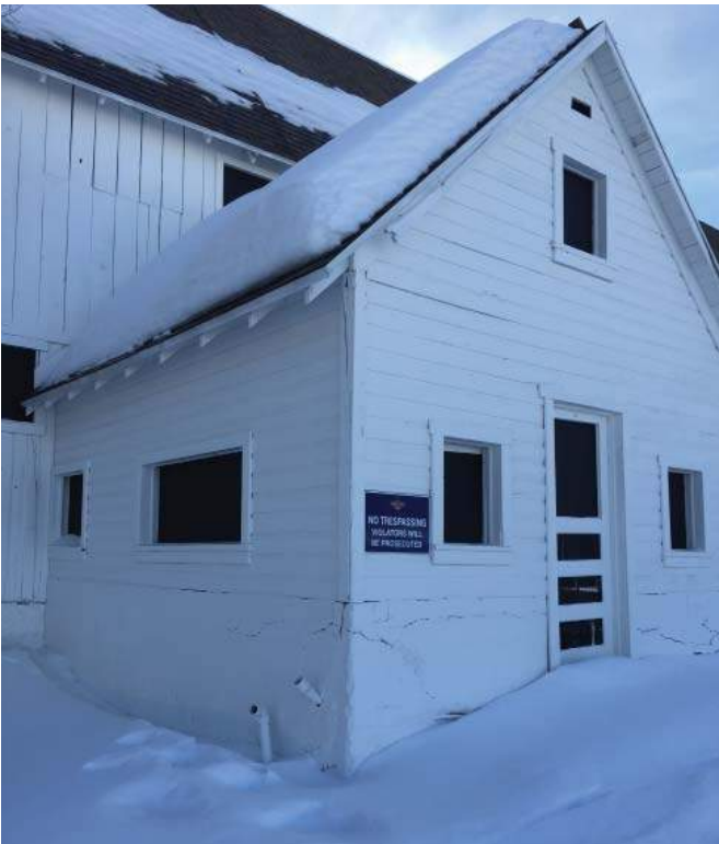
Photo #014: West Addition North and West Walls
