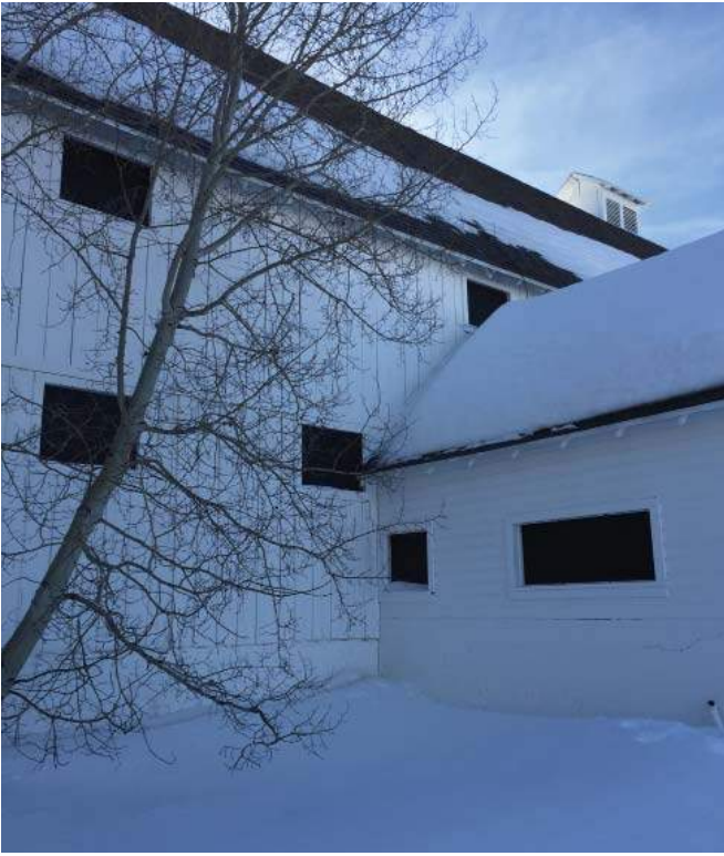
Photo #013: Barn West Wall / West Addition North Wall
