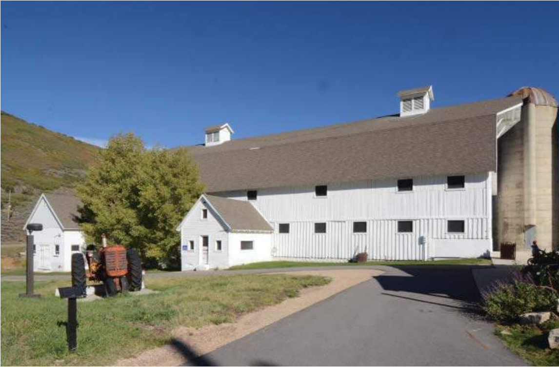
Photo #005: Roof from West
