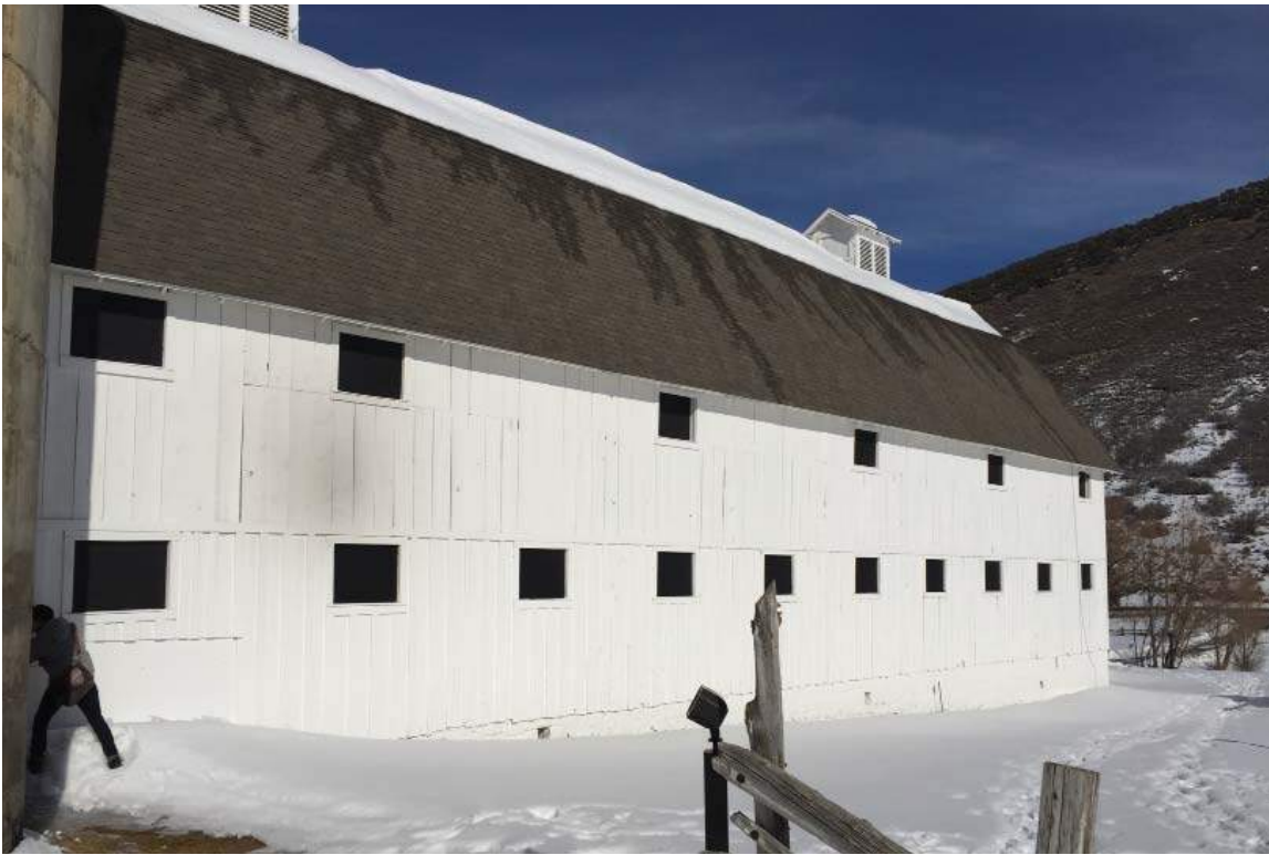
Photo #019: Barn East Wall
