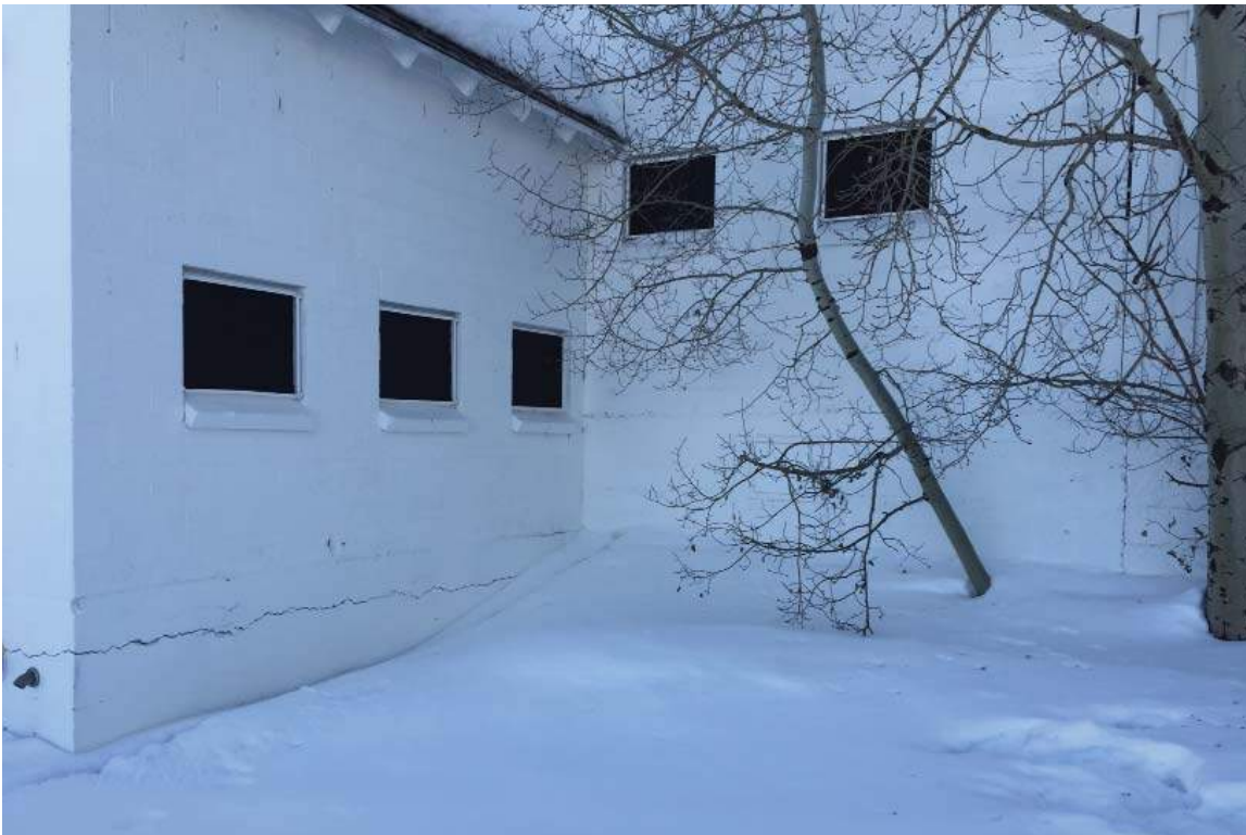
Photo #010: Northwest Addition from South
