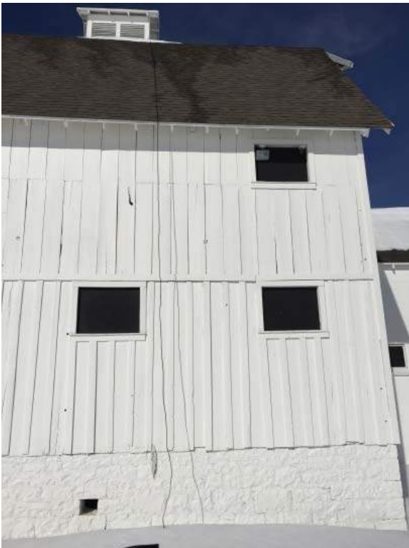
Photo #020: Barn East Wall
