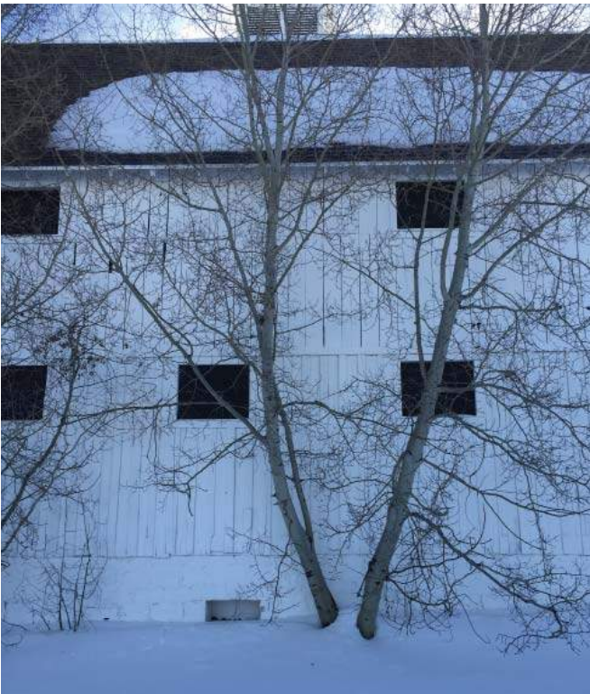
Photo #012: Barn West Wall
