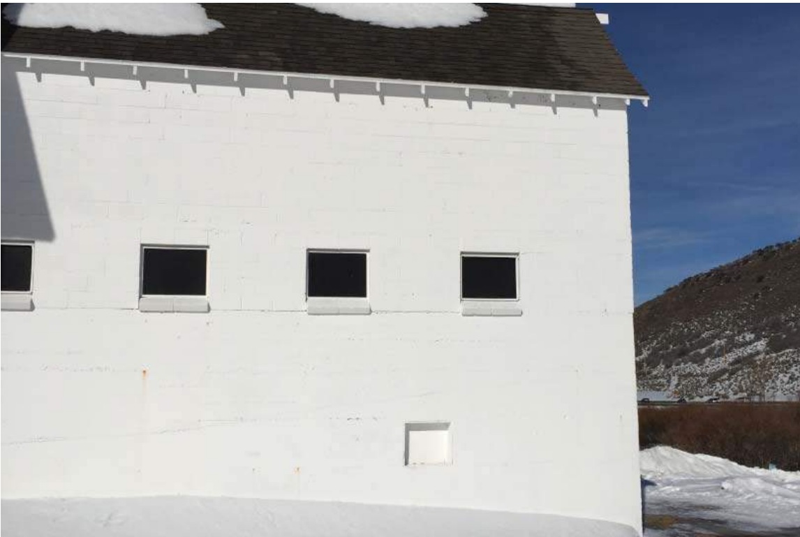
Photo #022: Northwest Addition East Wall
