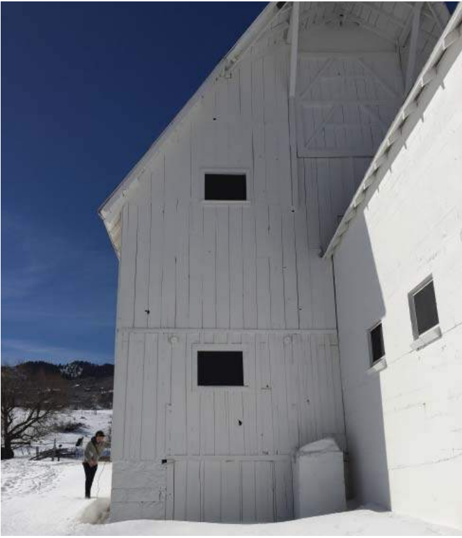
Photo #021: Barn North Wall
