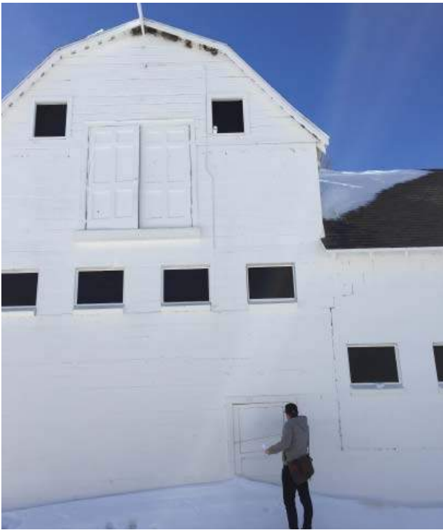
Photo #023: Northwest Addition North Wall
