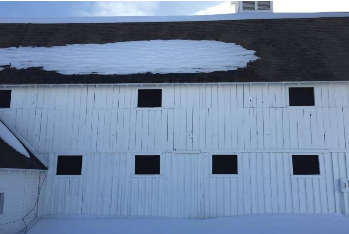
Photo #016: Barn West Wall
