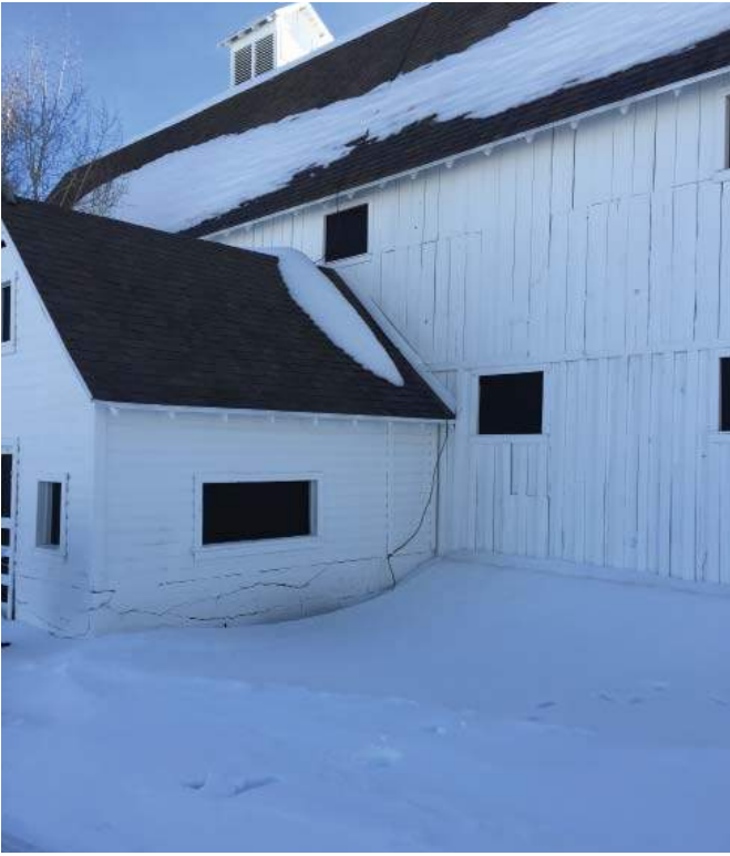
Photo #015: West Addition South Wall / Barn West Wall
