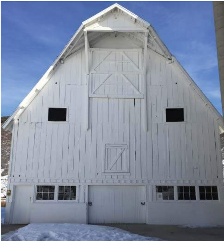
Photo #018: Barn South Wall
