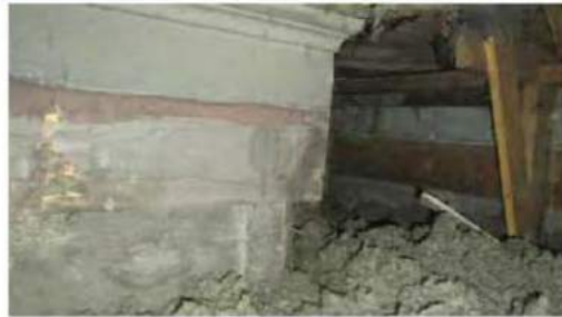
A5 HISTORIC FRIEZE AND FASCIA IS SHOWN AS IT ROUNDED THE FRONT CORNER OF THE HOUSE
