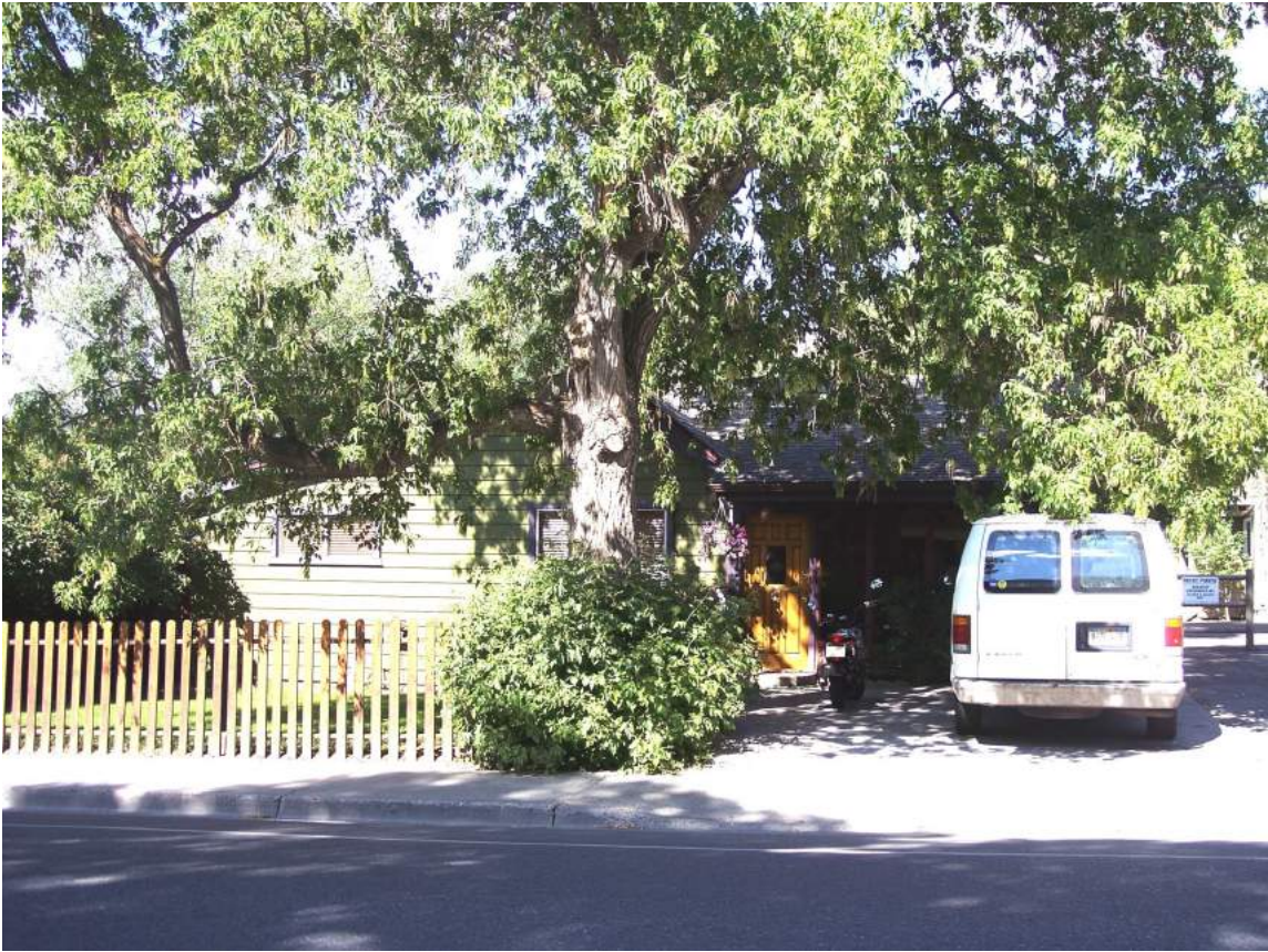
Photo No. 1: West elevation. Camera facing east, 2006.
