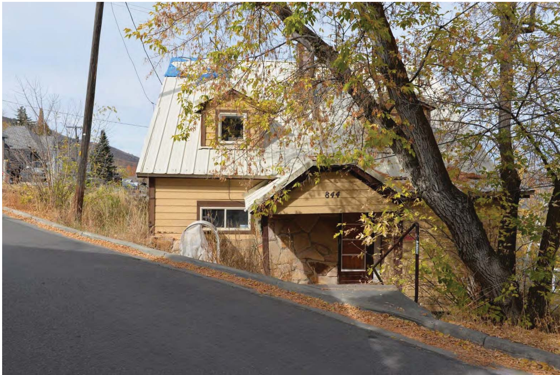
844 Empire Avenue looking northerly
