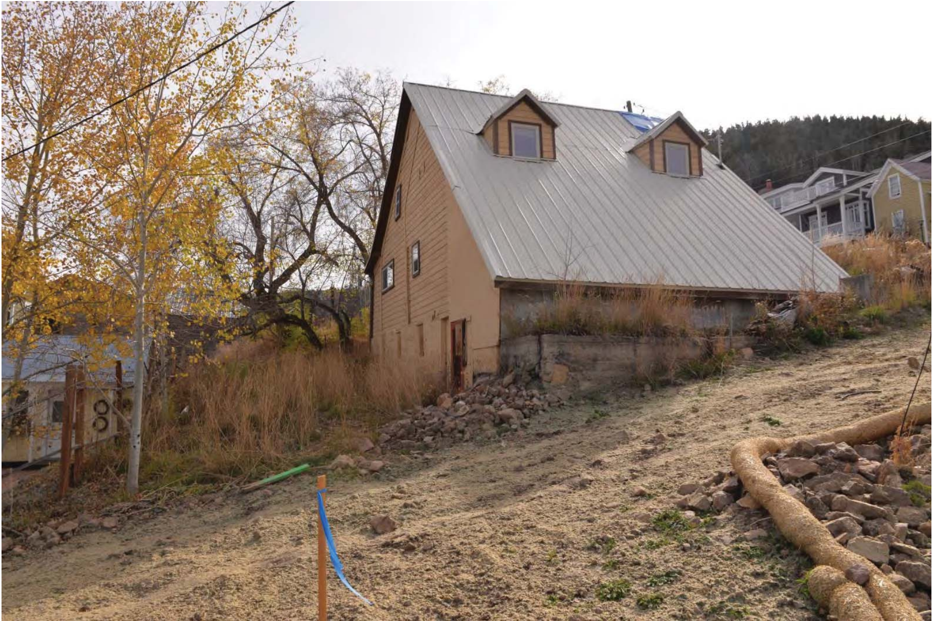
844 Empire Avenue looking southerly
