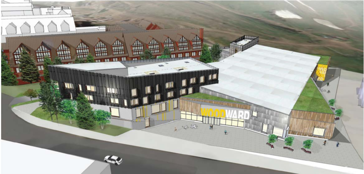
AERIAL VIEW TO SOUTHWEST ABOVE LOWELL AVE.
