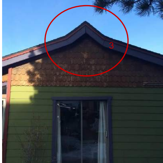
Photo of the south elevation, north-west wing.
