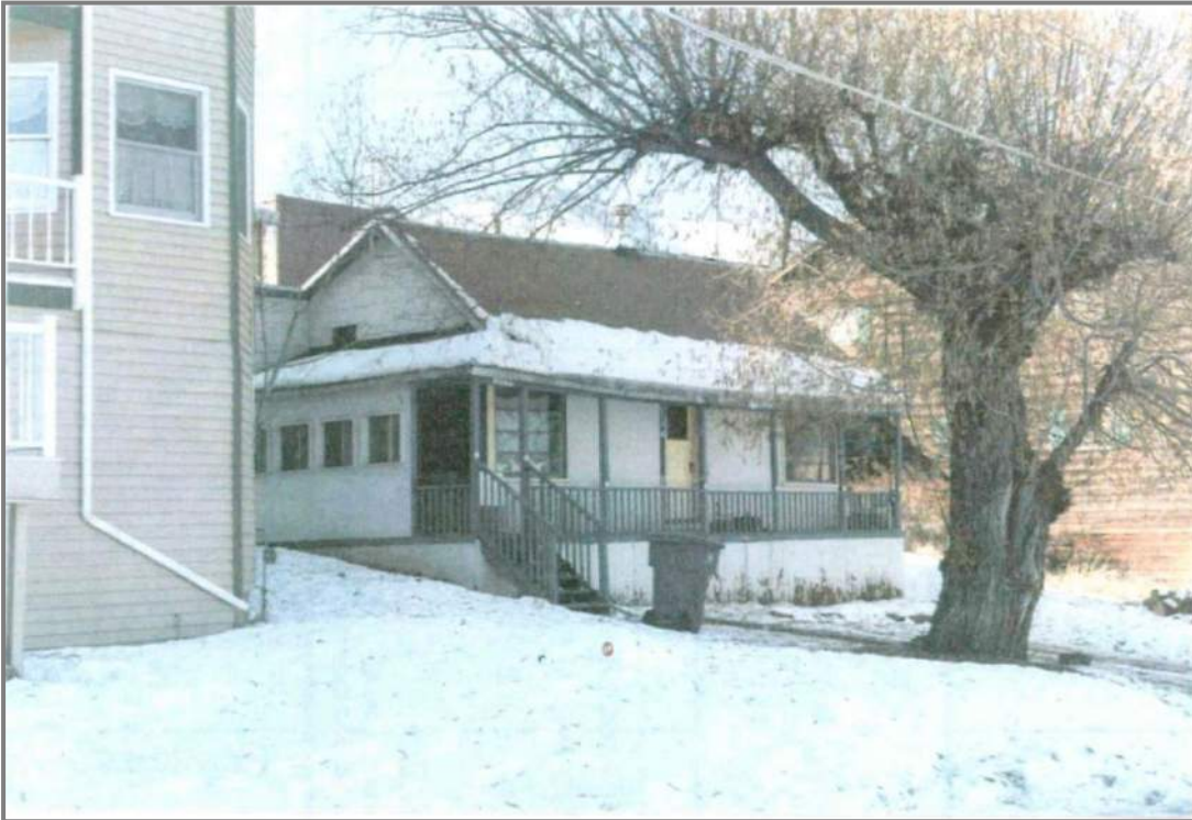
Figure 6: Southeast oblique. Camera facing northwest. 2001. Before the 2002 renovation.
