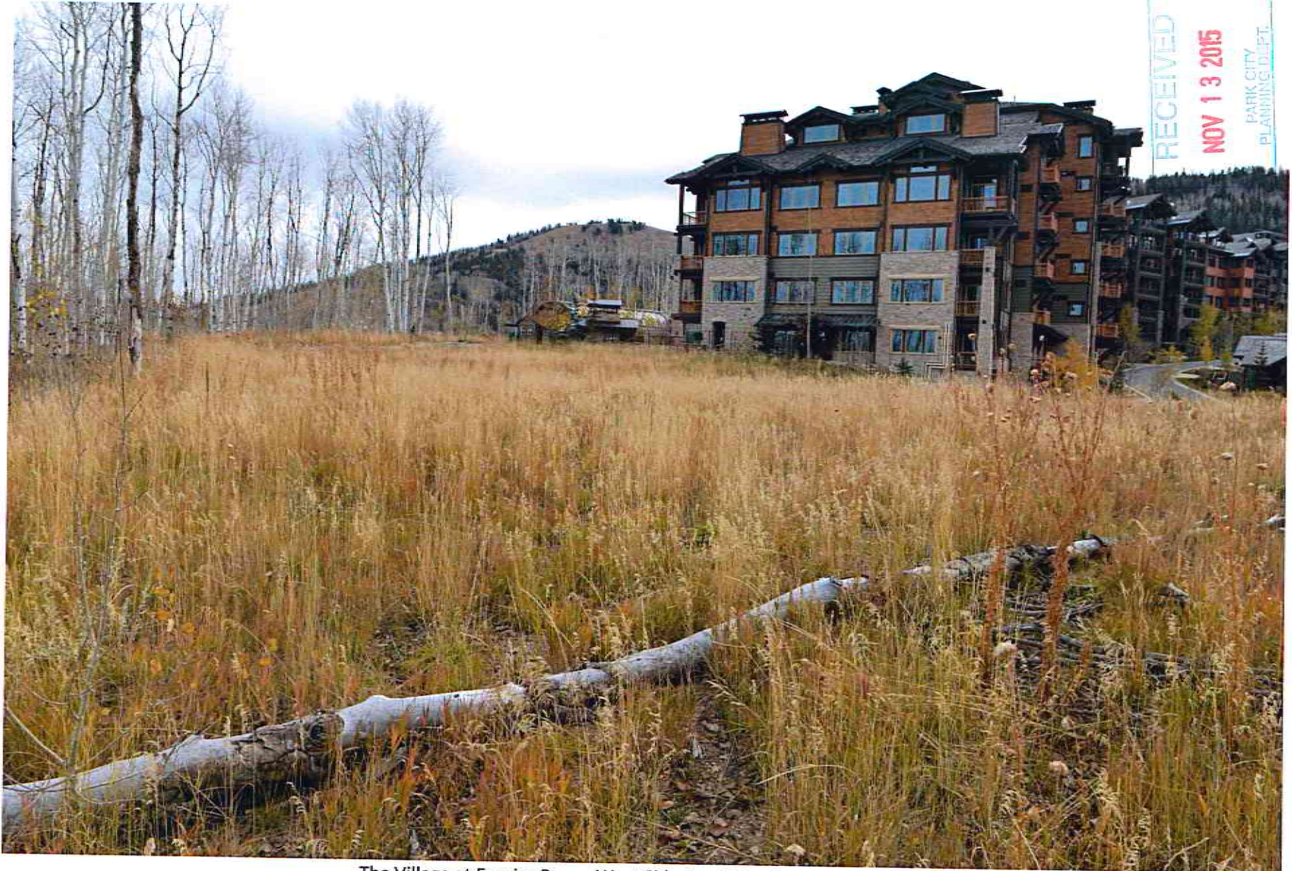
The Village at Empire Pass – West Side, Lot 15 looking southeasterly
