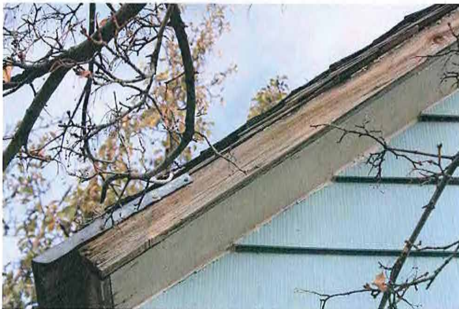
Soffit and fascia at northwest corner.
