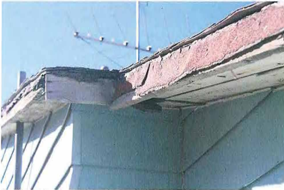
Soffit and fascia southeast corner kitchen/bathroom
