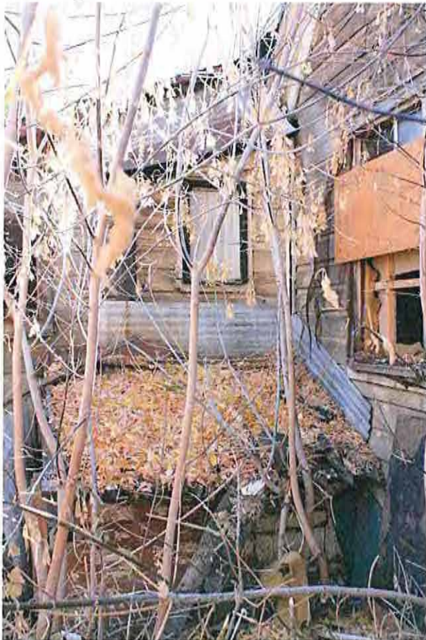
North elevation-shed access to mechanical
