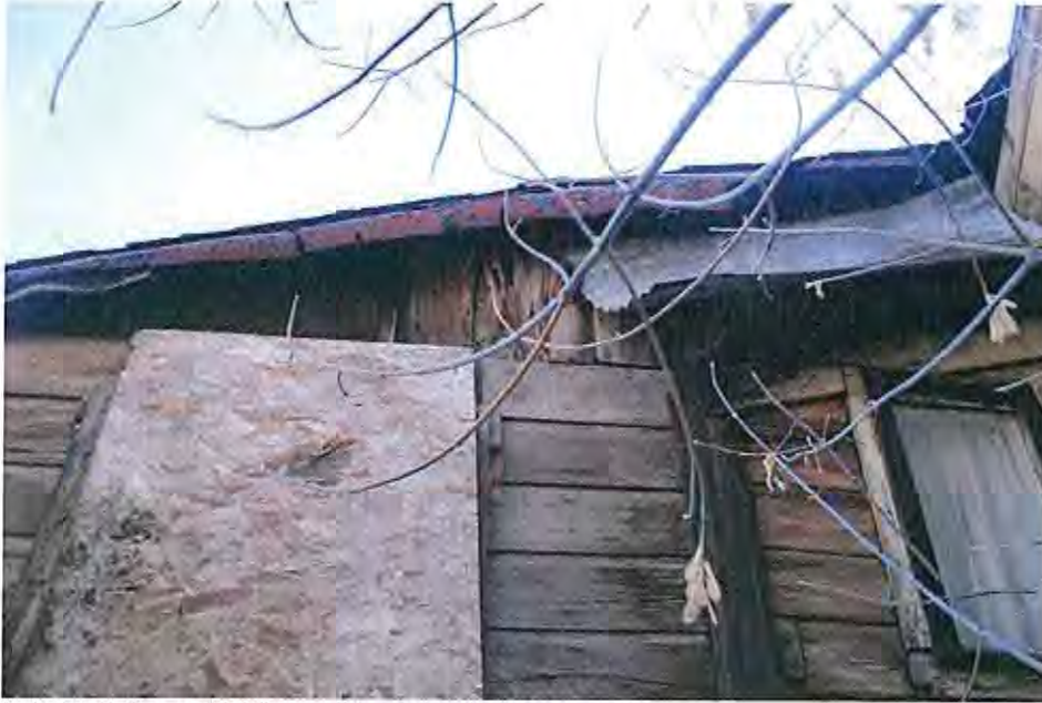
Intersection-sheds north elevation
