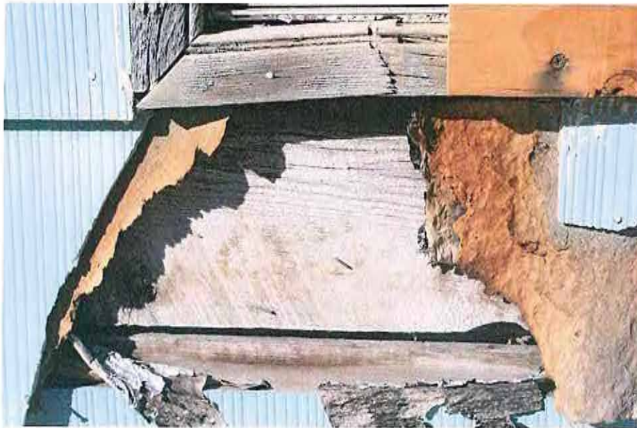
Typical 2" historic wood casing. This particular one is on the kitchen window.
