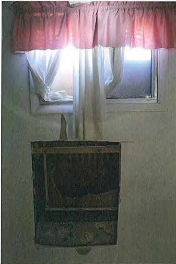
Interior east bedroom window
