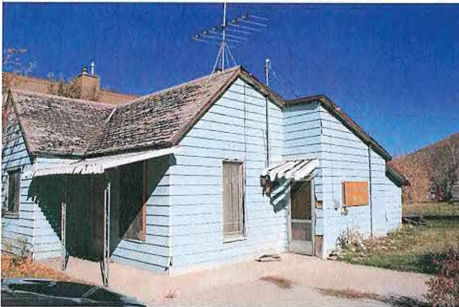
Intersecting cross gable roof with aluminum shed porch roof
