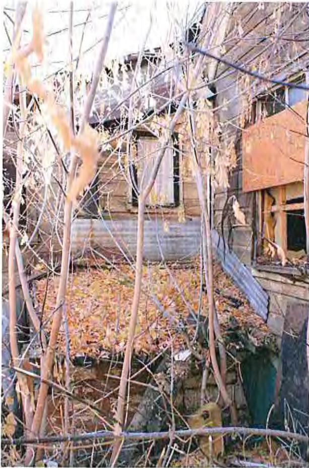
Northeast corner hole
