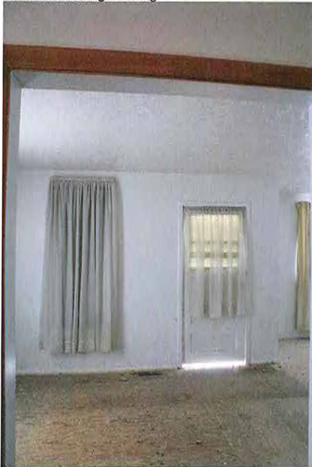
Ceiling lowered throughout house
