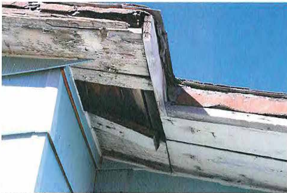
Detail soffit and fascia corner southeast 10"
