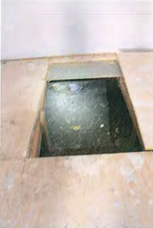
Dirt and rubble foundation-typical
