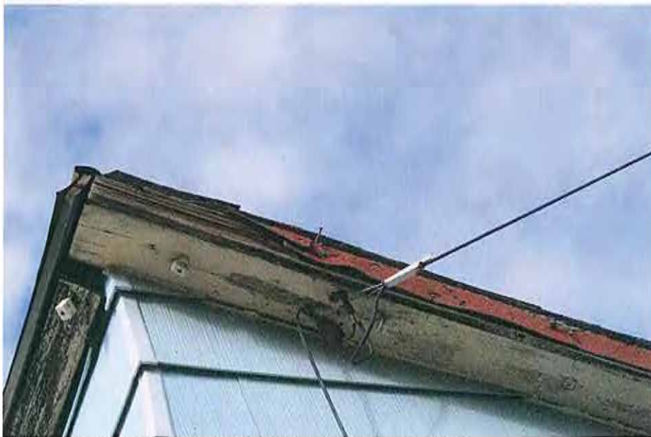
Overhang at west end of kitchen wall-south elevation
