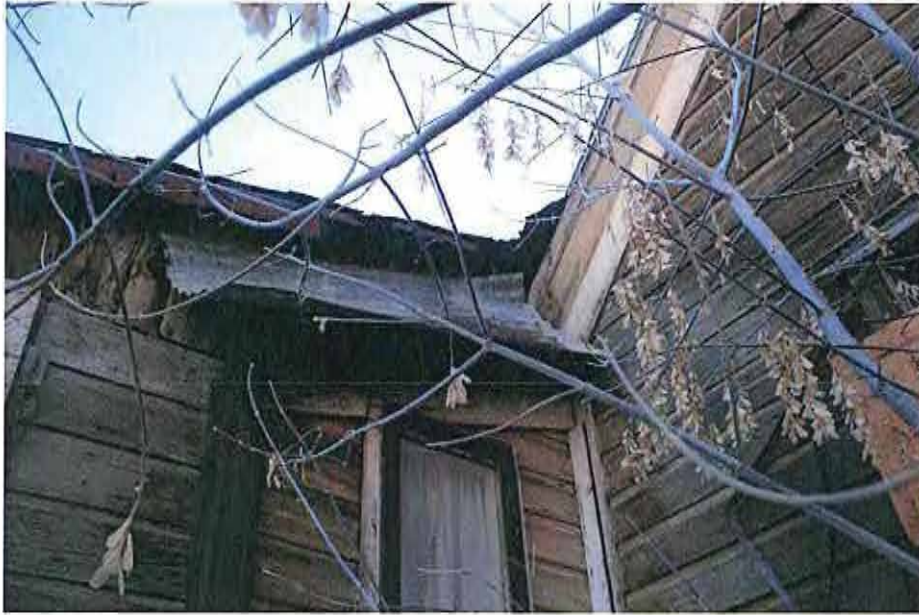
Corner- original 4'-0" shed structure
