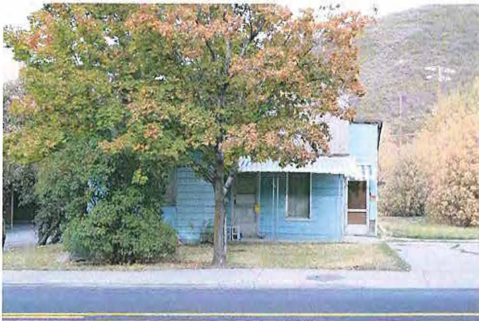
West elevation mature trees and vegetation-2010
