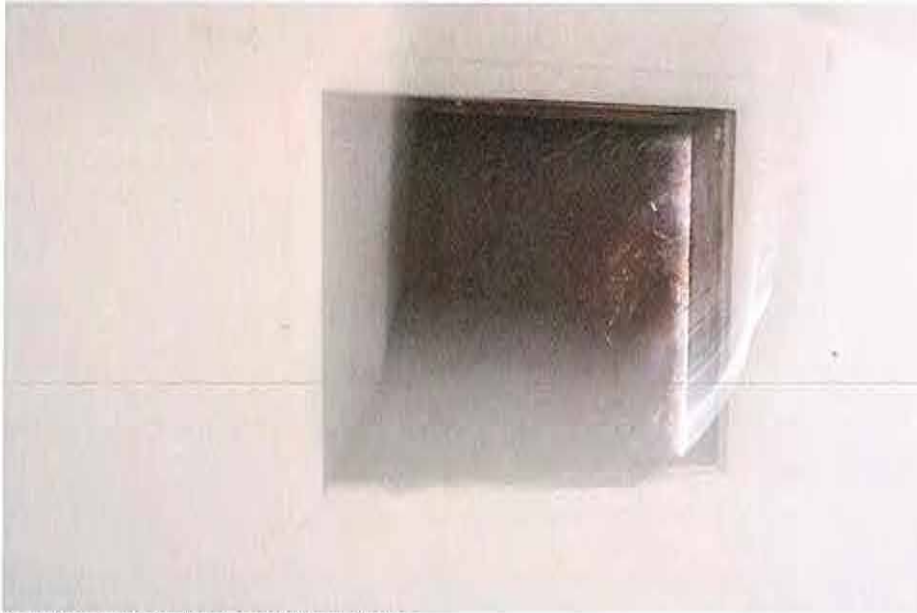
Northeast window-modified frame
