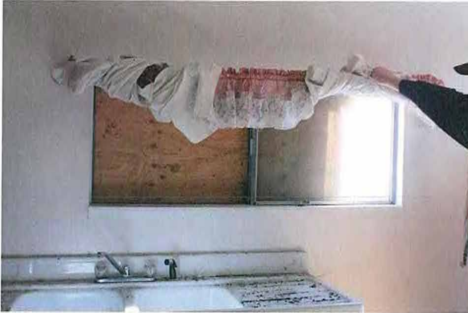
Interior kitchen window casing modified
