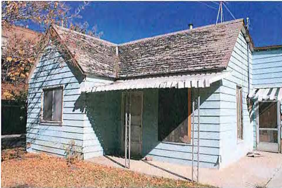
West primary façade- 2010 photograph
