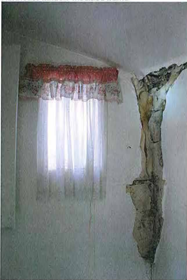
Interior northwest window
