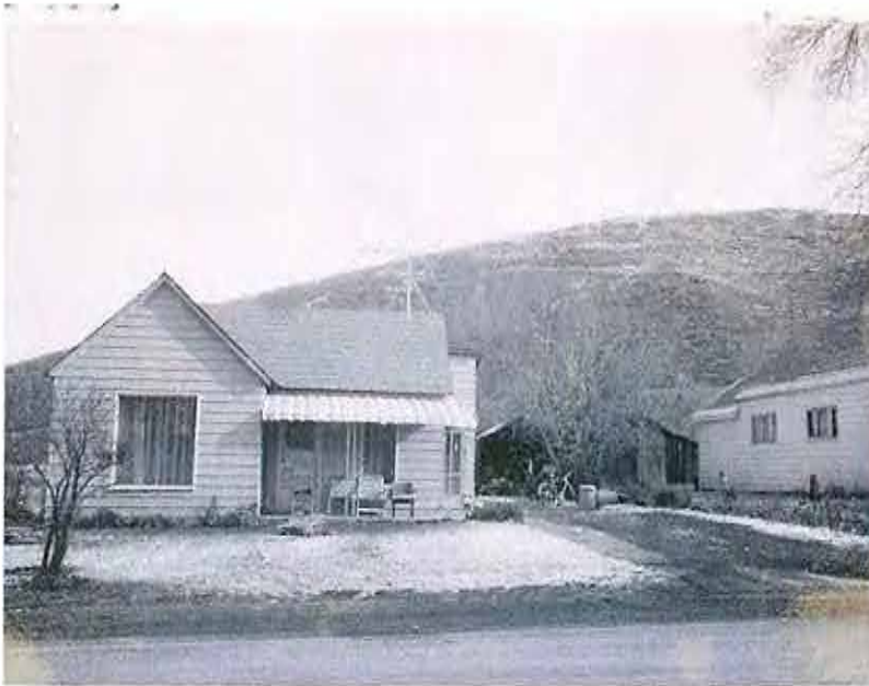
1958 photograph showing existing front door-possibly showing kitchen door as well
