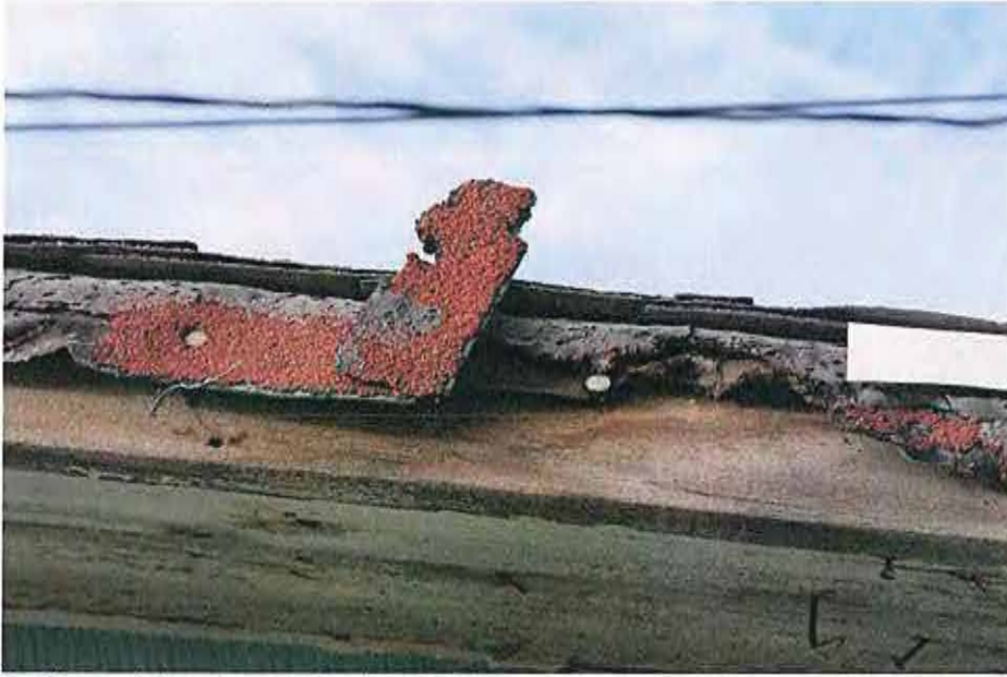
Soffit and fascia south elevation
