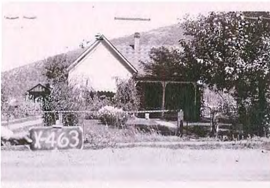
1450 Park Ave. Historic porch
