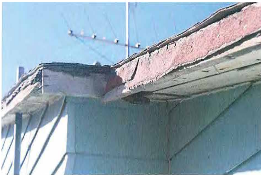
Transition from 6" overhang to 10" overhang
