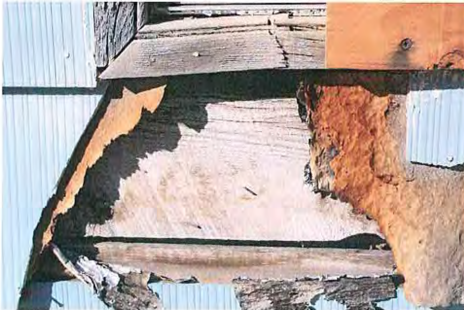
Typical 2" wood casing
