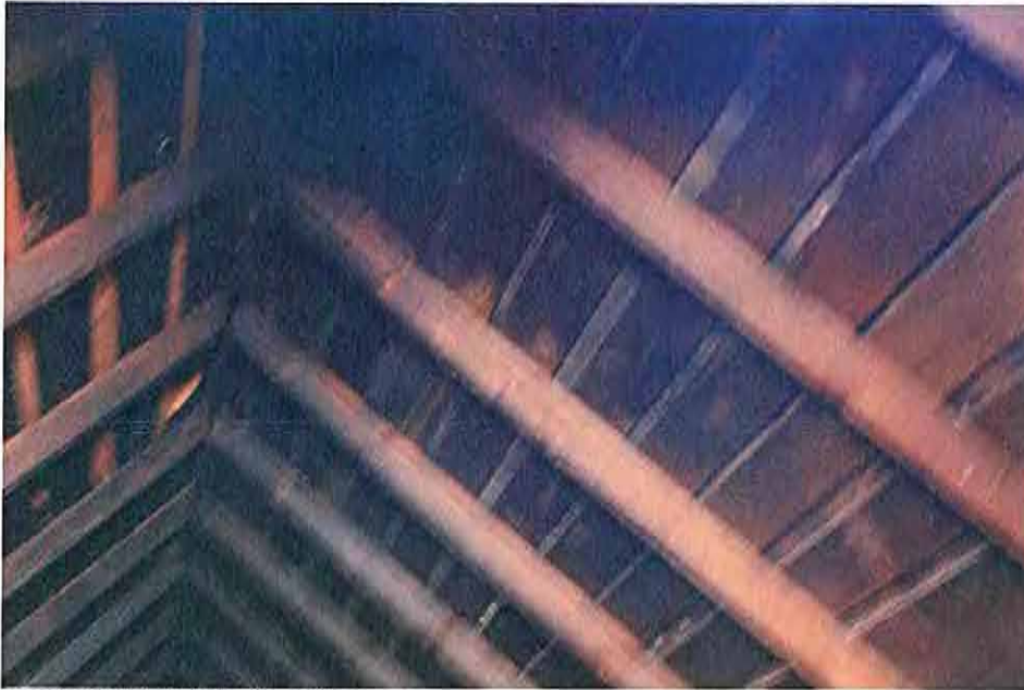
East-west gable framing
