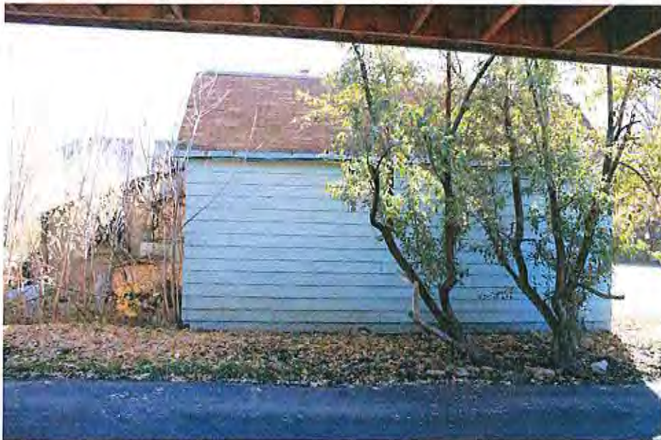
East-west gable roof
