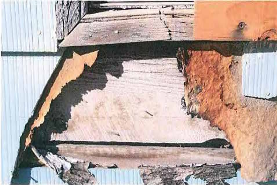
Exposed original wood lap siding, building paper, masonite, siding
