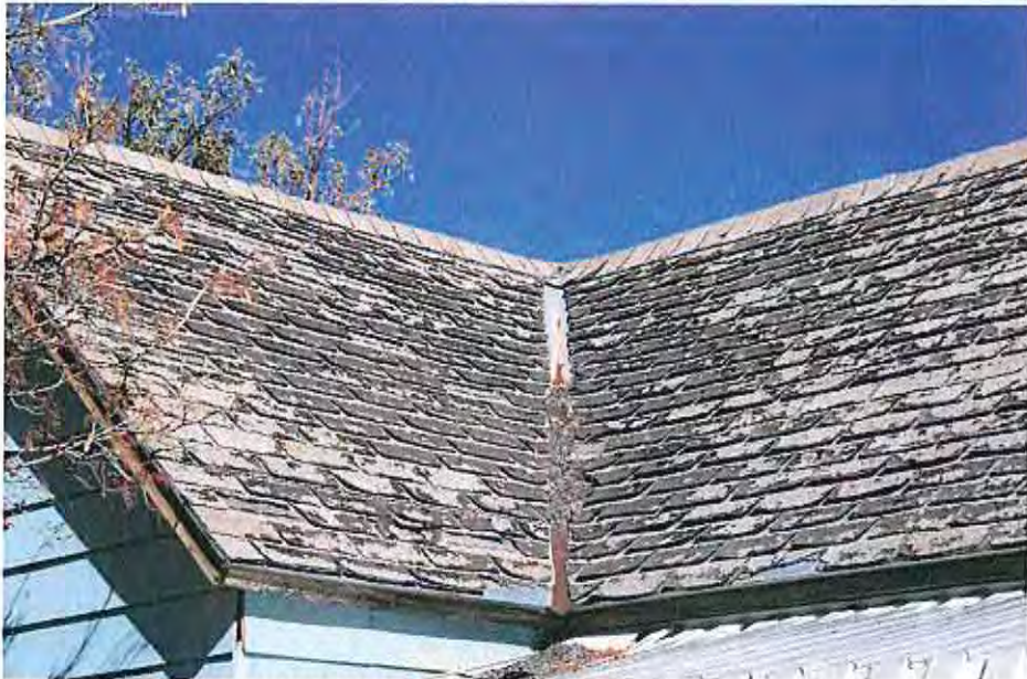
Intersection-valley east-west gable and north-south gable
