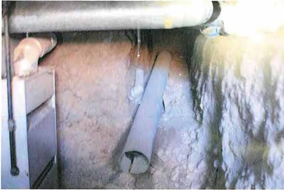
Duct work through excavated dirt
