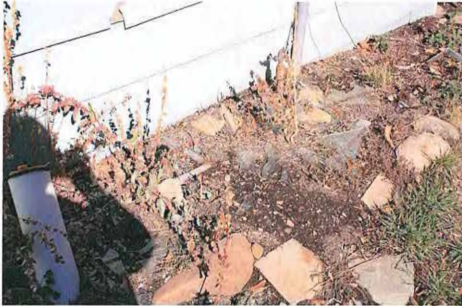
Water turn off, hose bib, and sink venting
