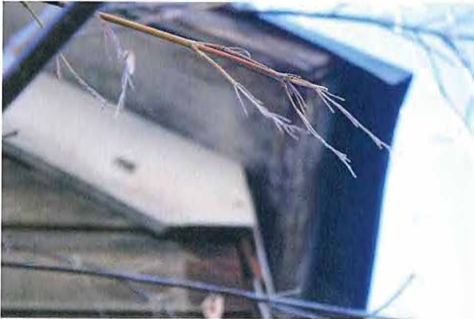
Original soffit, fascia and trim. Sheet metal drip edge.
