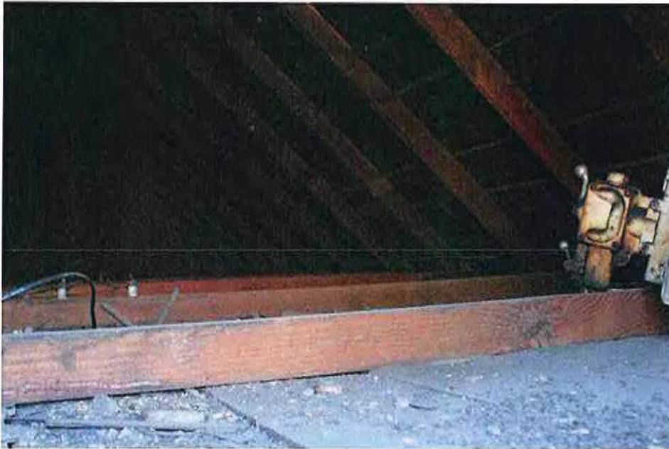
Roof and ceiling framing
