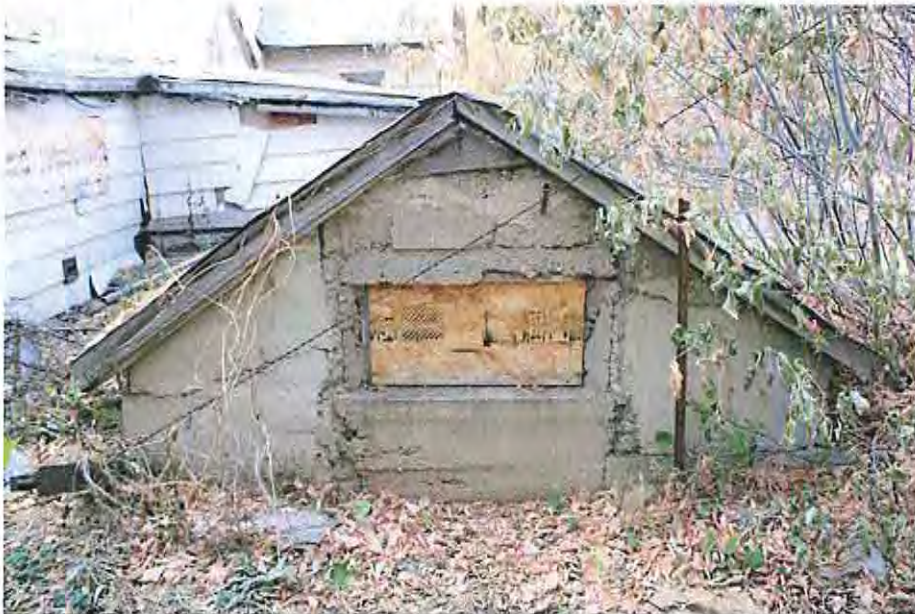
South elevation-root cellar
