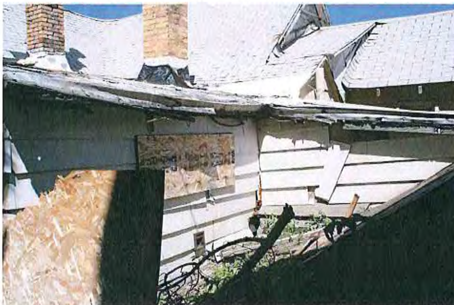
This is a double hinged, single pane window manual casement window on the east side of the mechanical room. It is 2'-10" off the ground and is 4'-6" W (2@ 2'-3" each) X 1'-5"H. There is a similar window in the small east bathroom gable.
