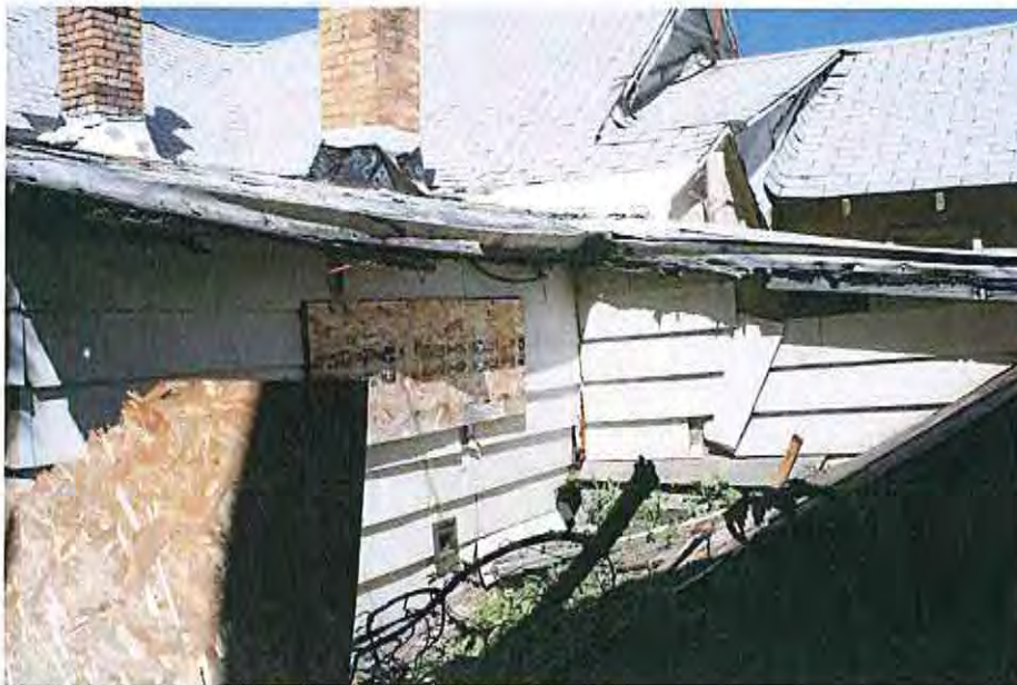
2. East elevation mechanical room shed
