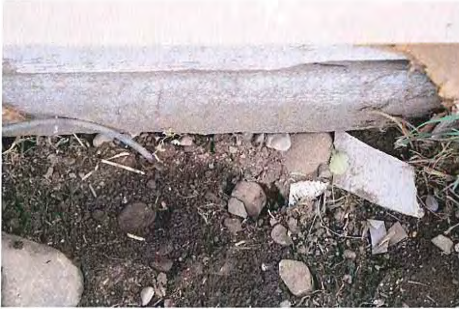
1.Foundation rubble-north elevation
