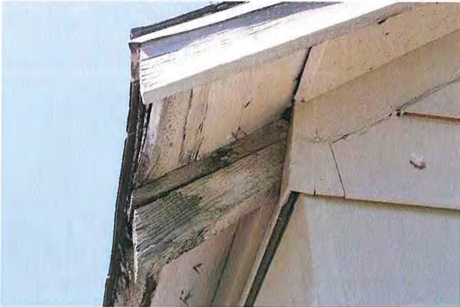
5.Soffit and fascia northwest corner
