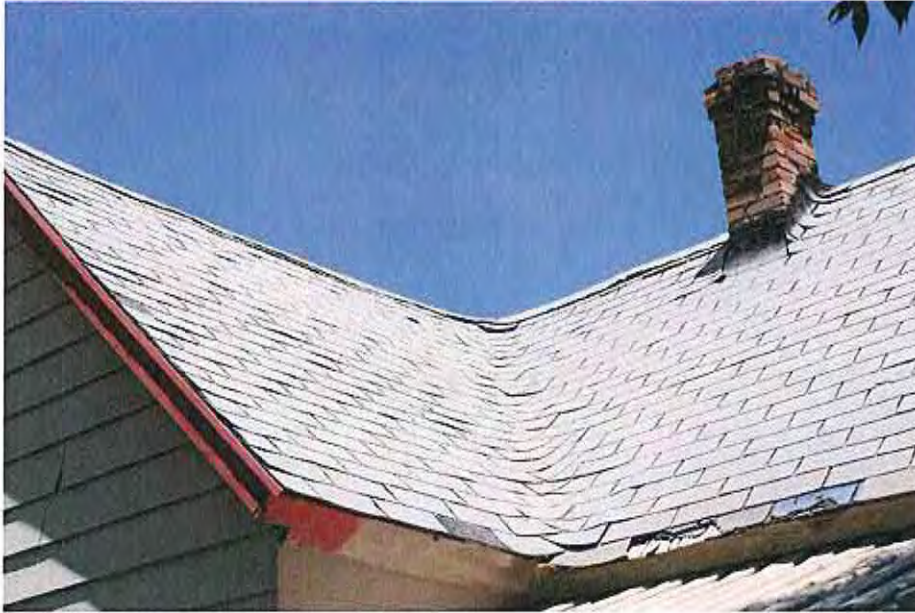
4. Original roof valley and chimney
