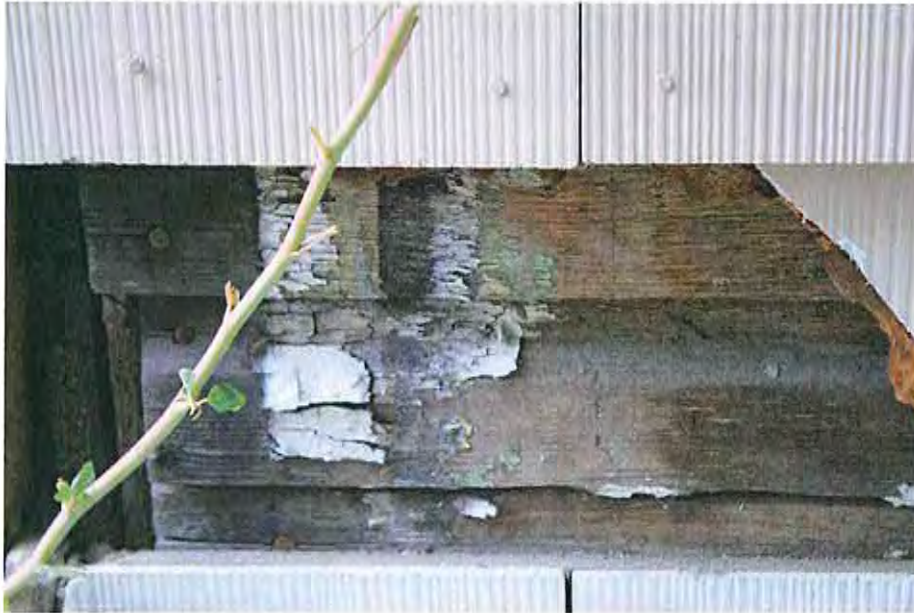
2. Siding detail northwest corner
