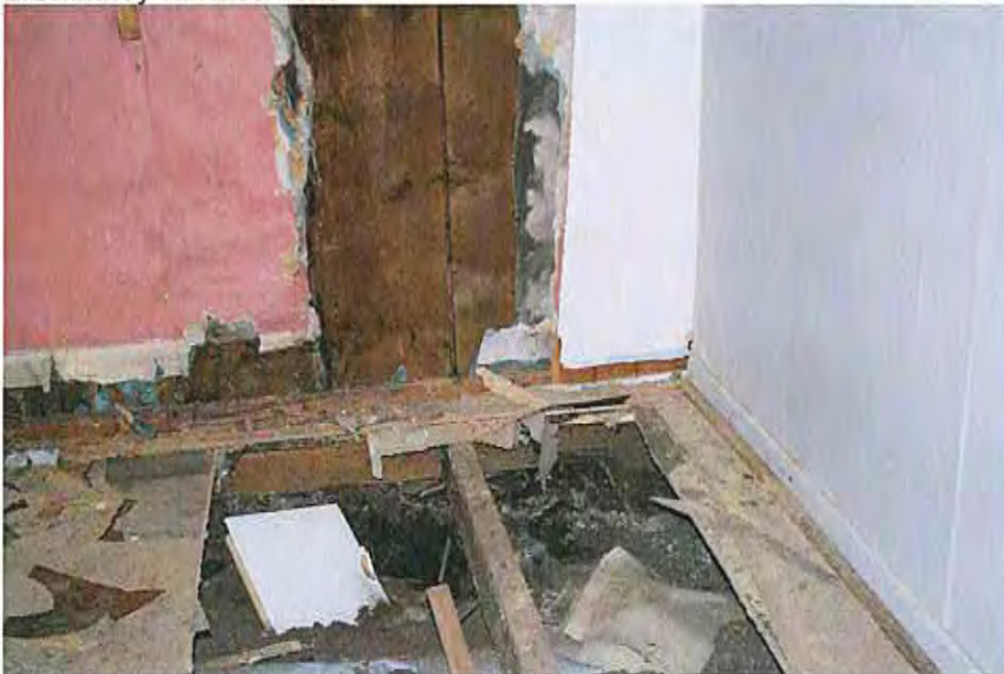
3. Duct work in foreground under floor joist
