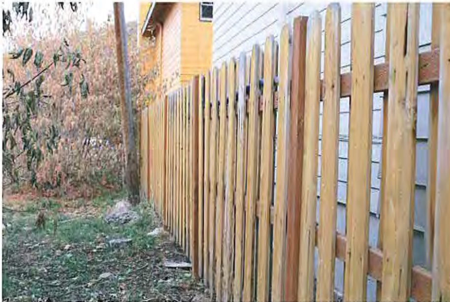
1.South property line wood fence
