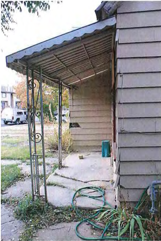
3. Porch- south elevation
