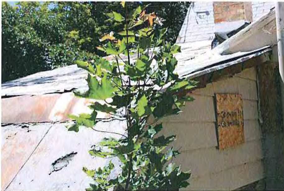
Window at stair to root cellar.
