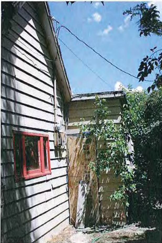
5. West kitchen door
