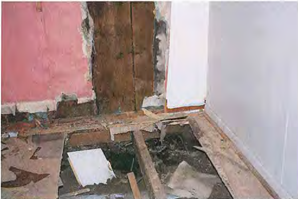
1. 1X12 wall construction. 2 1/8"X6" floor joist.
