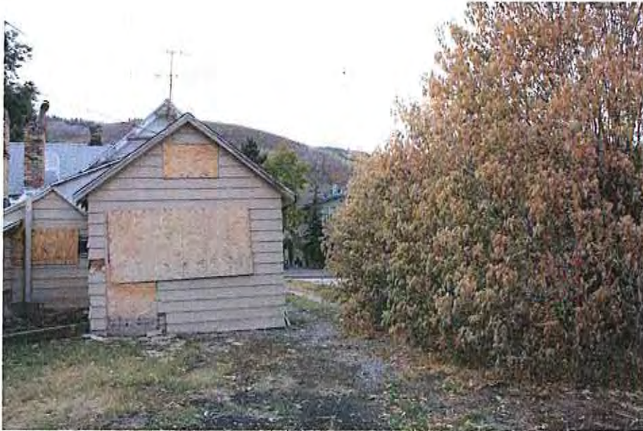
5. Northeast gable-north façade
