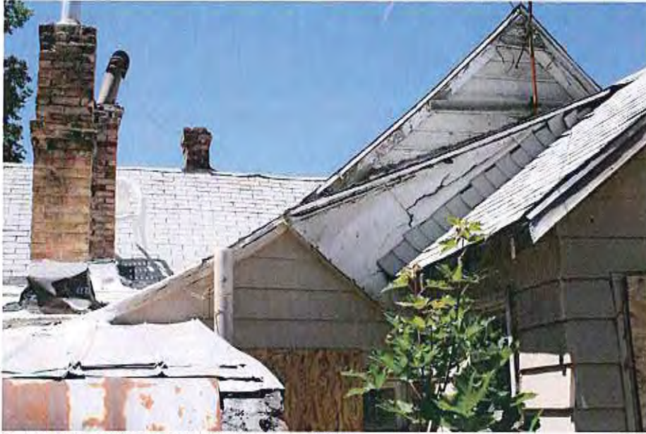
3. East elevation-small bathroom gable
