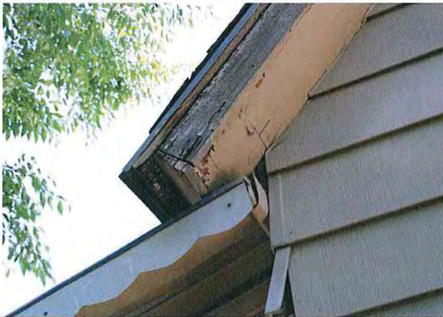
3.Original south gable roof and porch roof intersection
