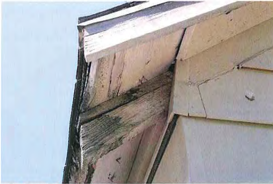
2.Soffit detail northwest corner
