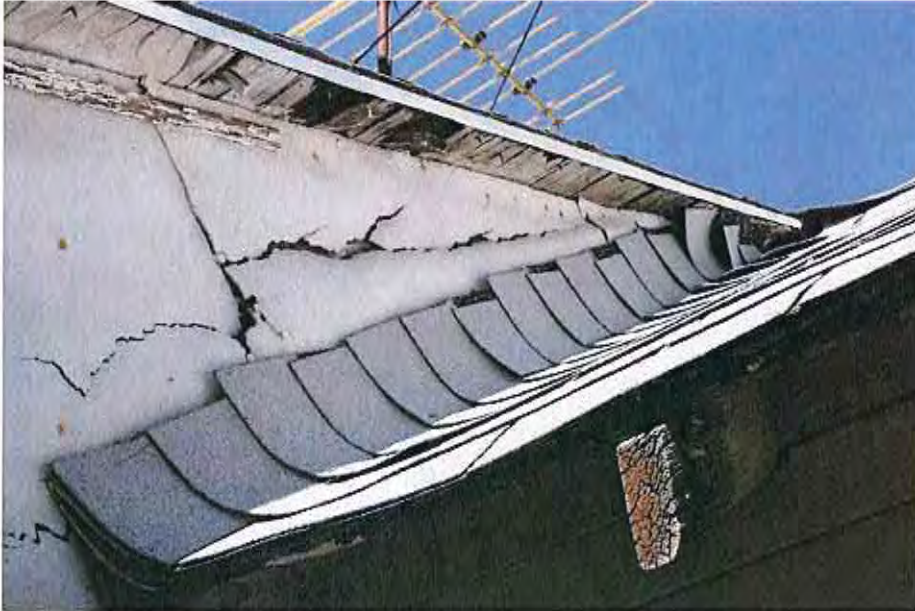
6. East elevation overbuild at bathroom
