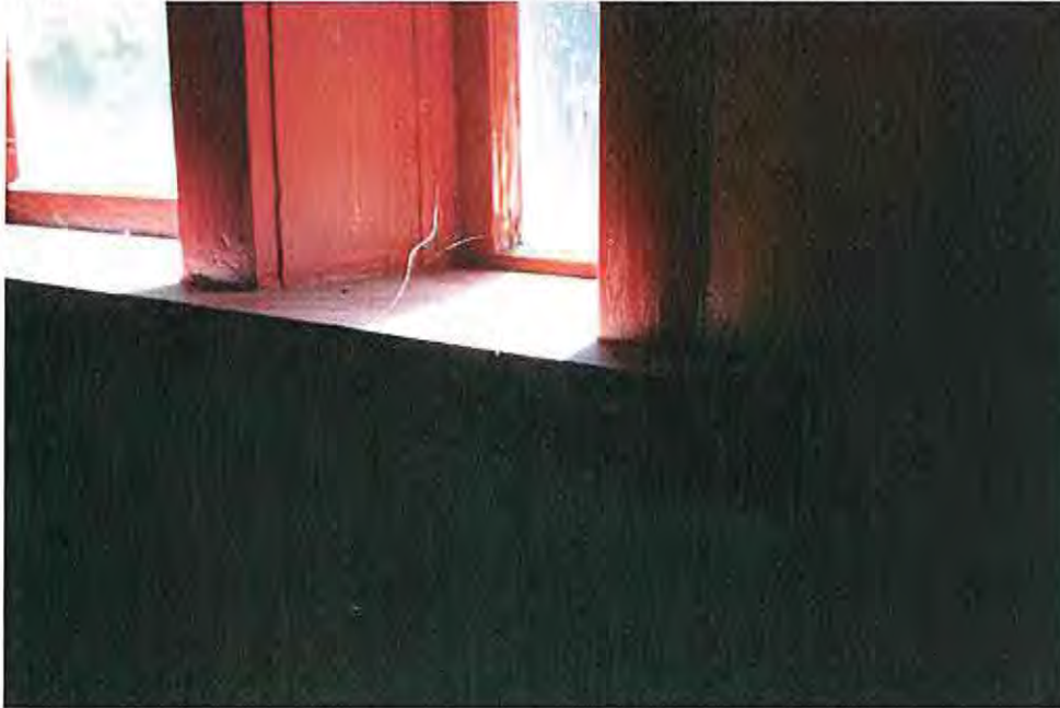
Interior of window detail.
