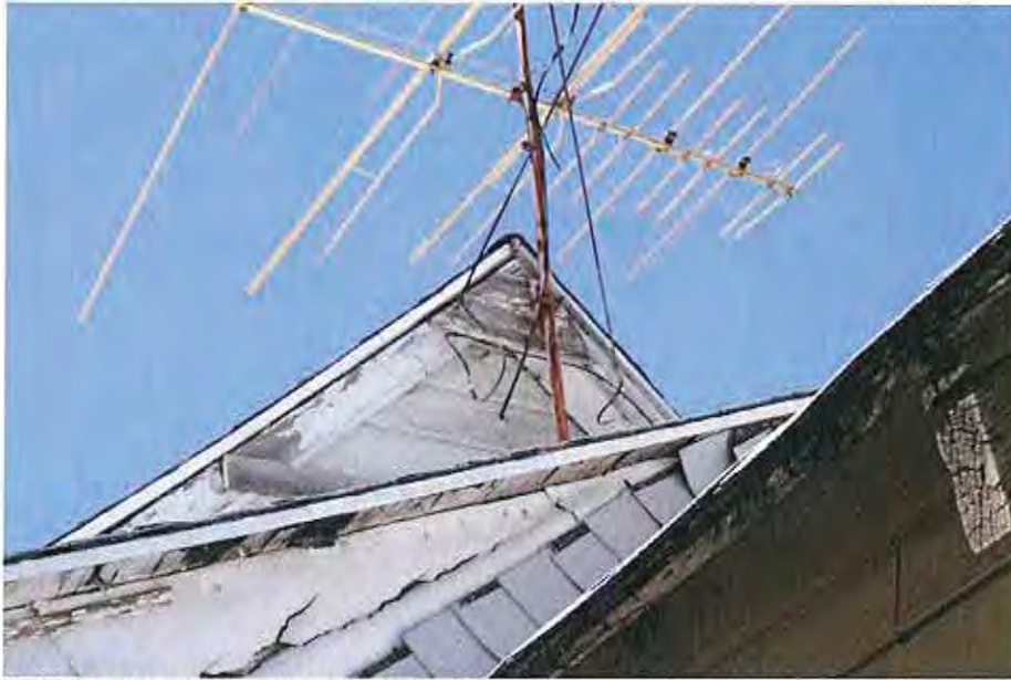
7. East elevation- original east/west gable
