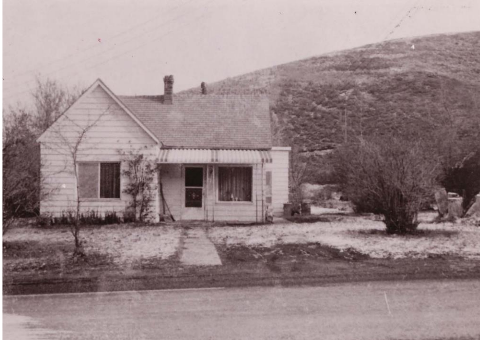
This c. 1958 photograph shows the new kitchen addition, which exists today. It also shows the new asbestos siding, metal porch, and the modifications to the window openings on the front façade.
