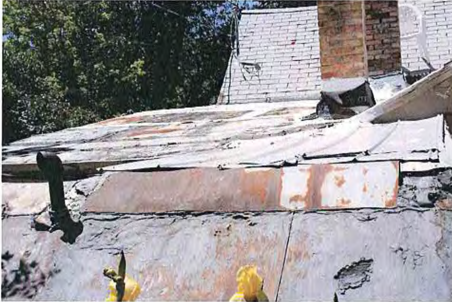
8. East elevation roof condition and chimneys
