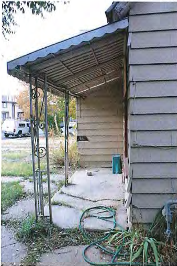
1.Original porch intersection-southwest corner
