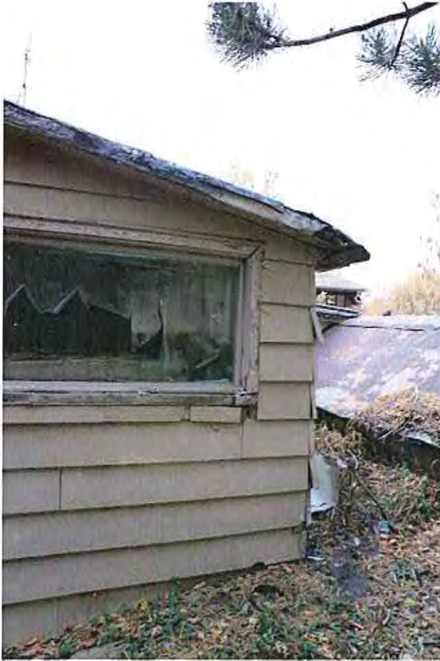
5. Southeast corner mechanical room
