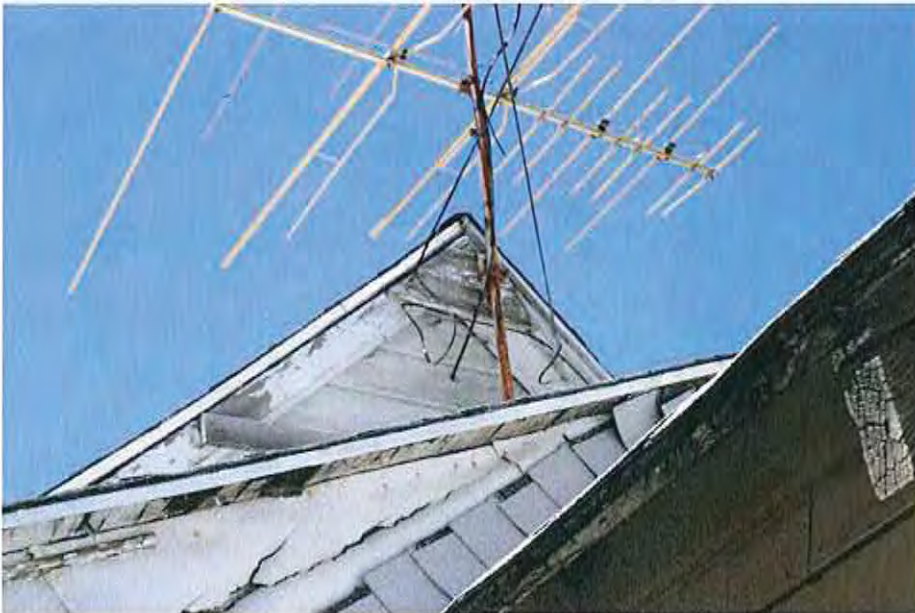
5. East elevation original gable
