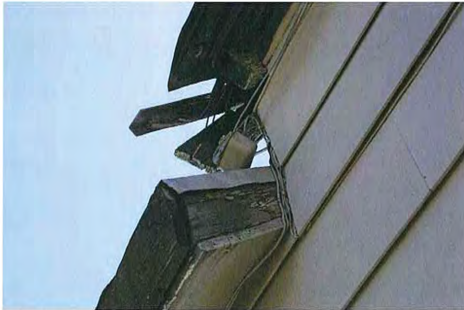
4.Soffit and fascia north elevation intersection original and addition
