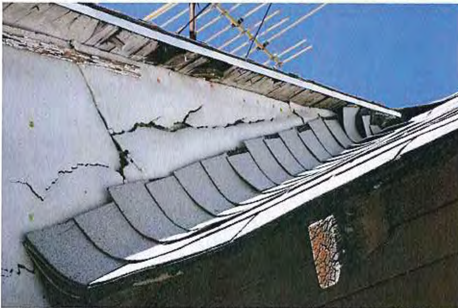
4. East elevation-extension overbuild to northeast gable from small gable
