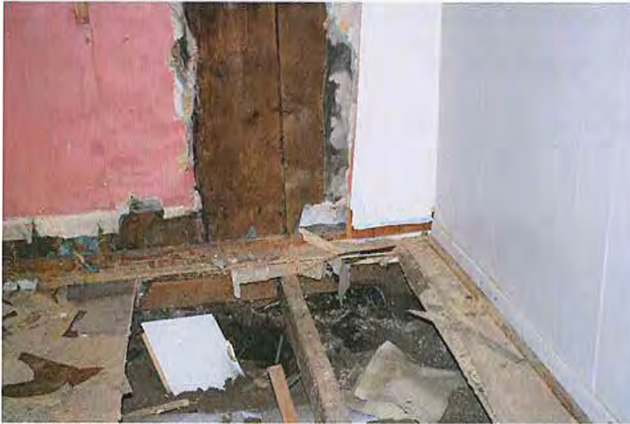
1.Look at interior excavation north wall
