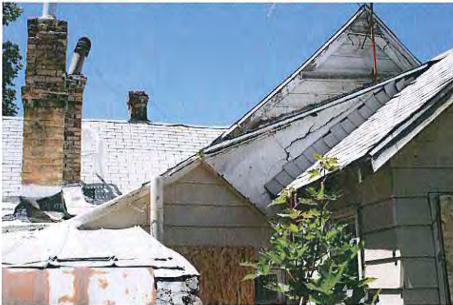
7. Toilet plumbing vent.
