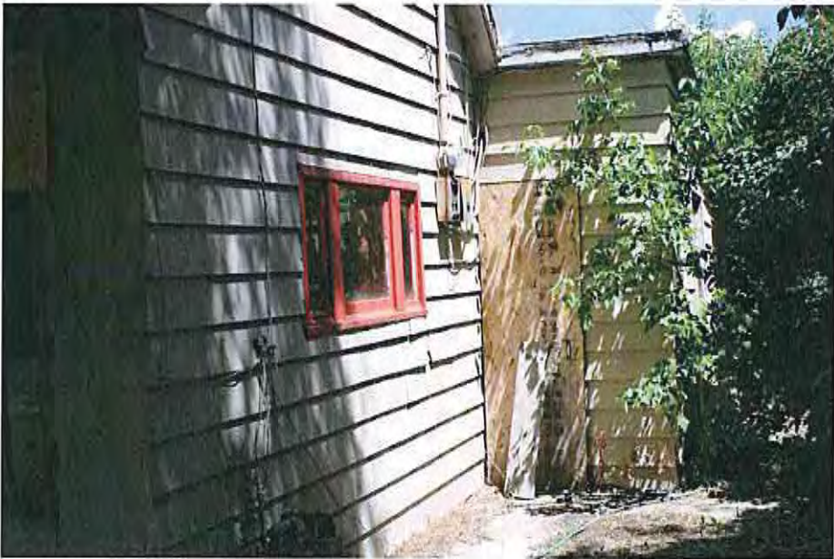
3. South original gable with electrical drop and gas meter
