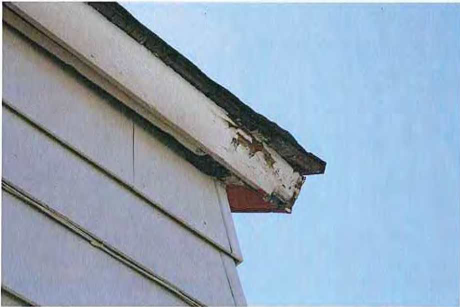
6.Fascia detail northeast corner
