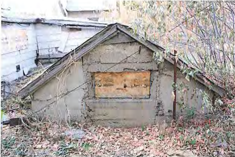
7. South elevation root cellar
