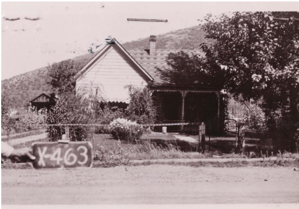
This photograph, taken c. 1938 shows the original porch and wood siding. The awning above the window would have been added in the 1920s-1930s, and hides the original window configuration of the front gable.
