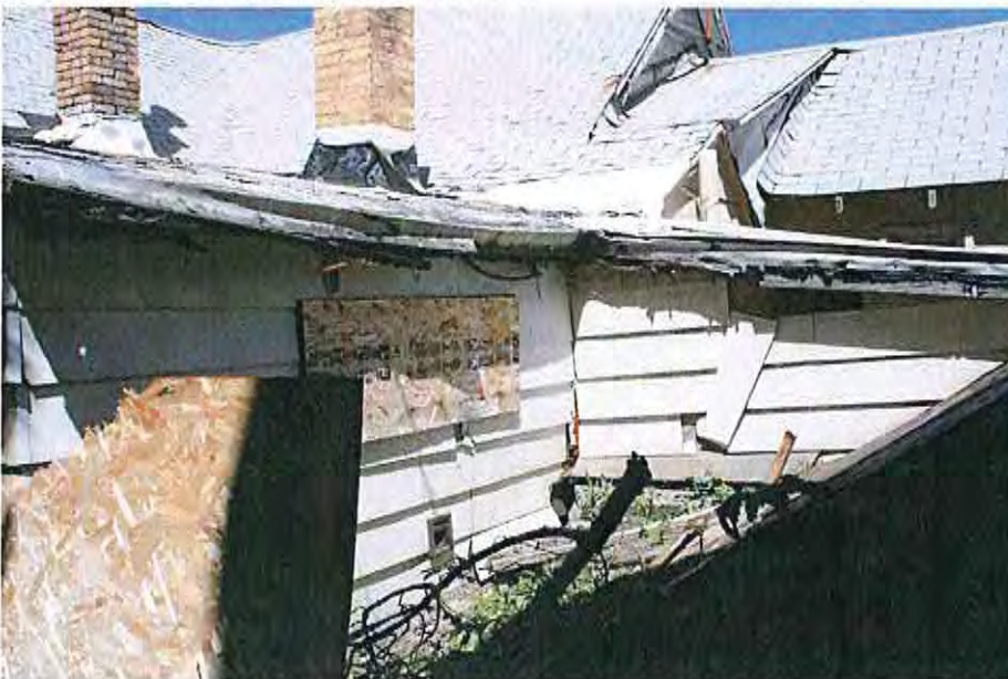
6. South elevation space between mechanical and root cellar. Covered stairs to root cellar to north.
