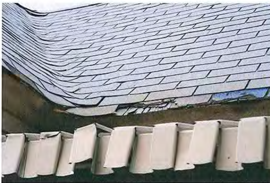
1.Original wood shingle
