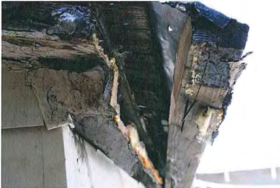
7. Fascia at southeast corner
