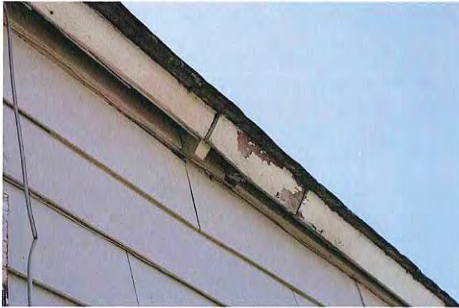
3.Fascia north elevation
