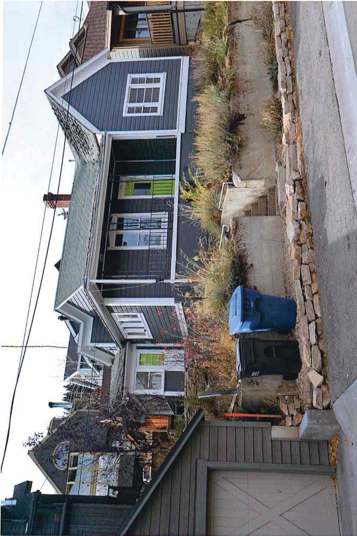
823 Norfolk Avenue looking westerly
