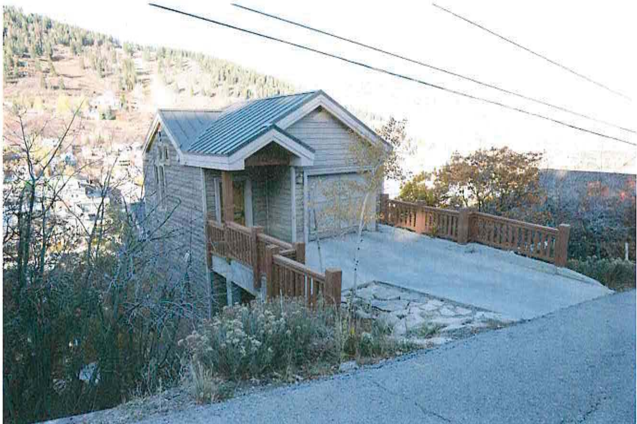
347 Ontario Avenue looking west
