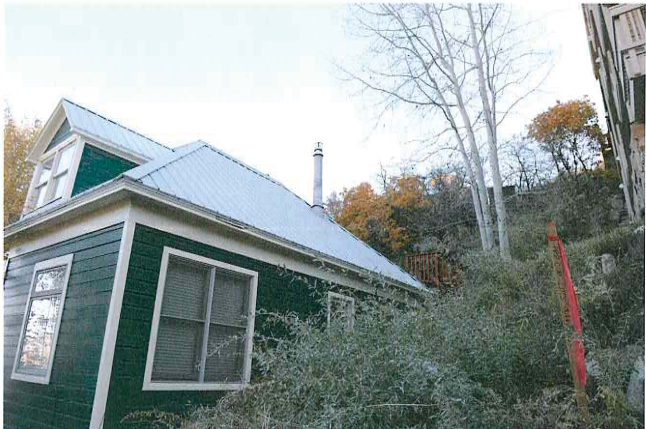
355 Ontario Avenue looking east
