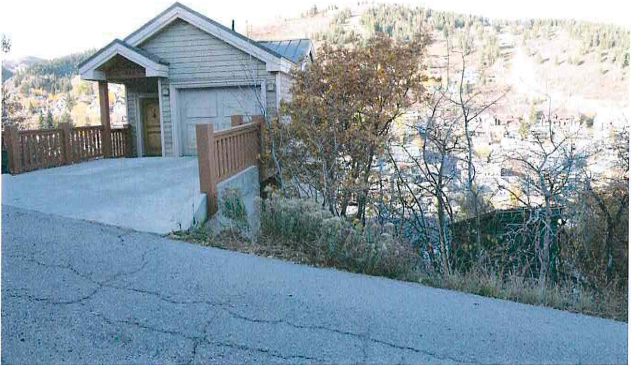
347 & 355 Ontario Avenue looking west
