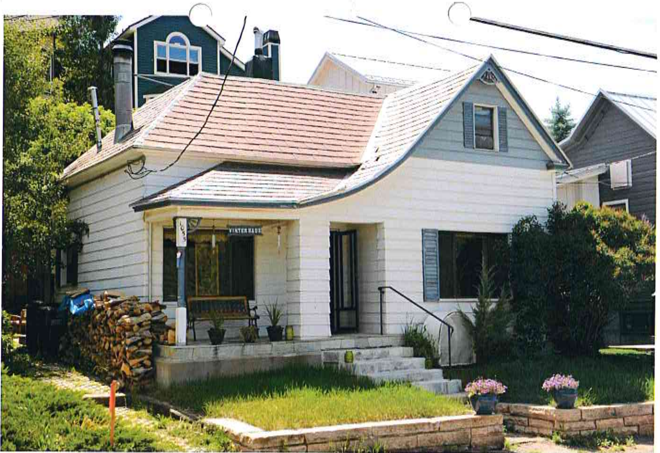
1055 Norfolk Avenue – Looking westerly
