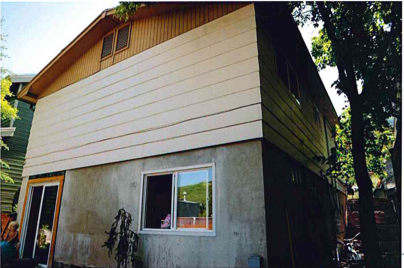
812 Norfolk Avenue – Looking westerly
