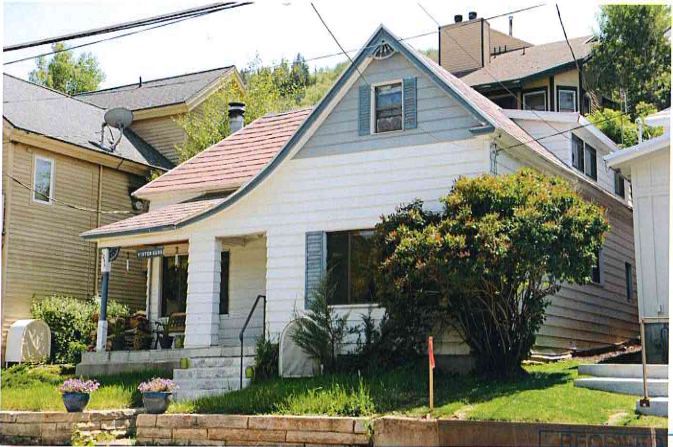
1055 Norfolk Avenue – Looking westerly
