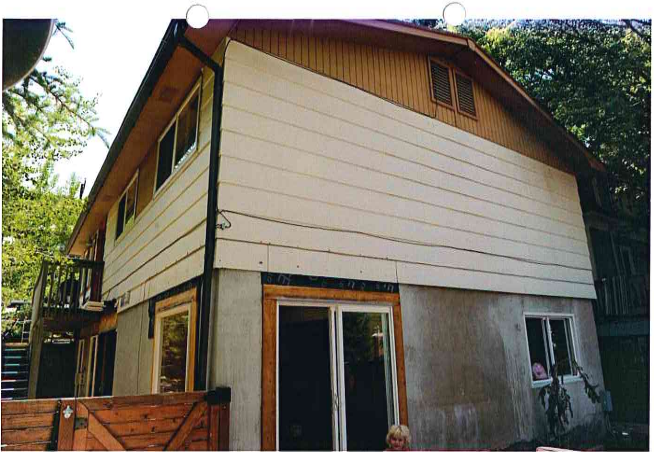
812 Norfolk Avenue – Looking westerly
