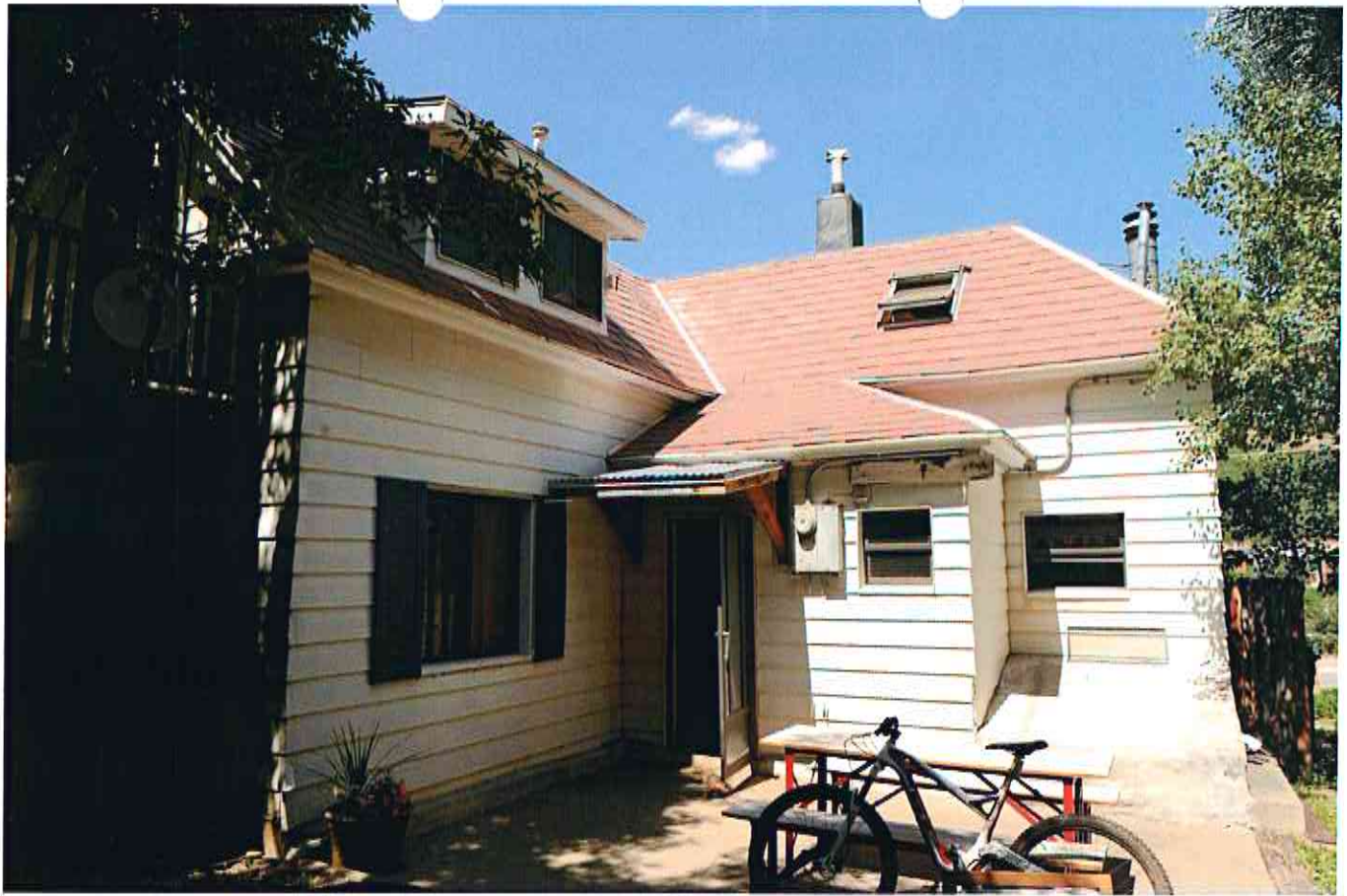
1055 Norfolk Avenue – Rear looking easterly
