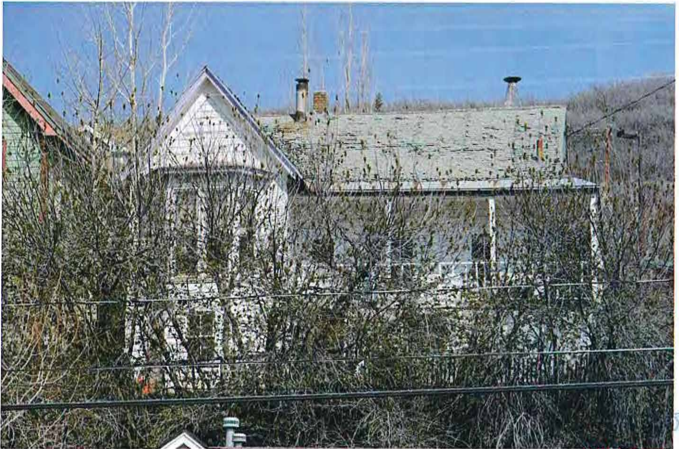
222 Sandridge Avenue looking East
