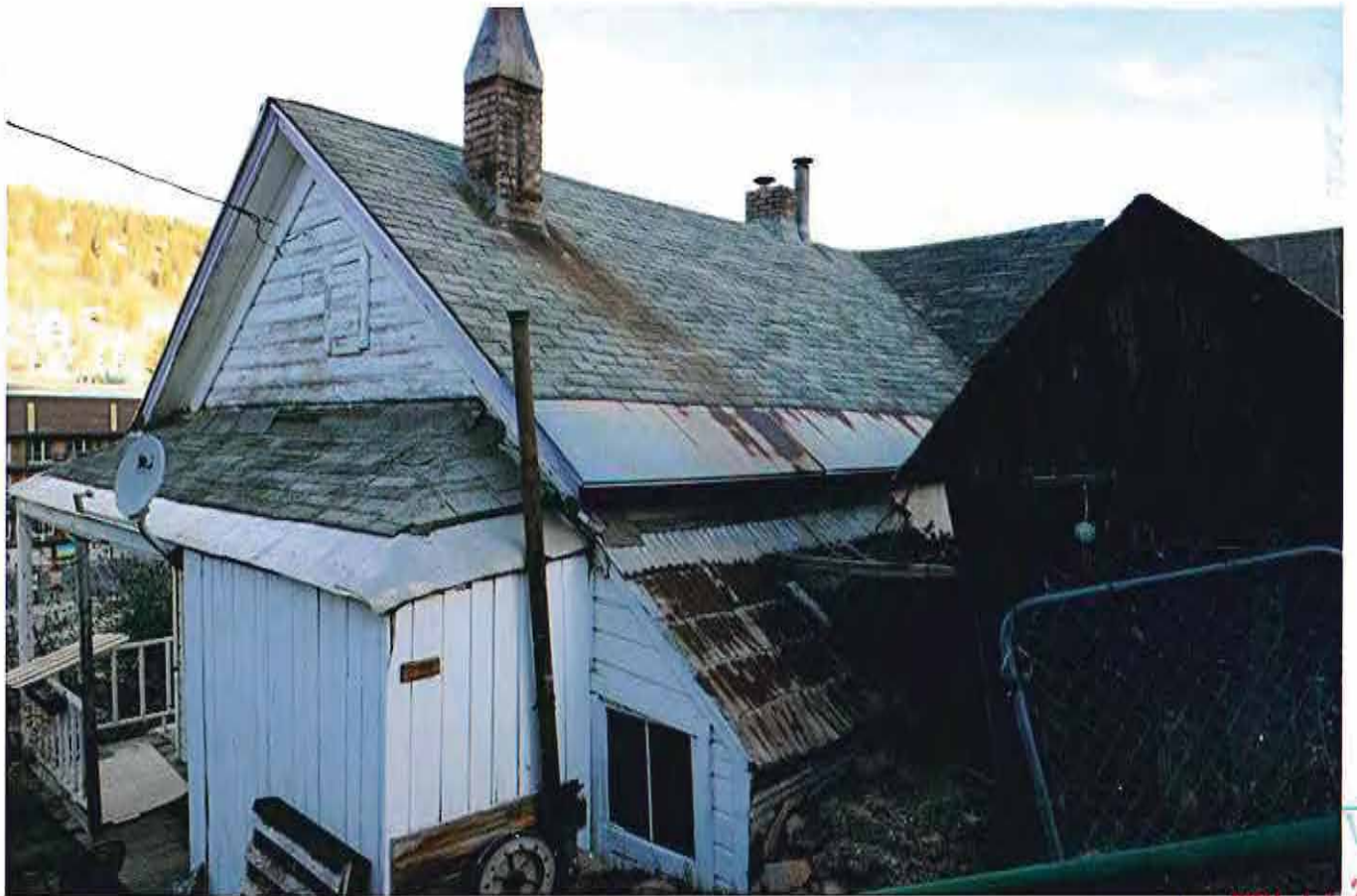
222 Sandridge Avenue looking Northwest
