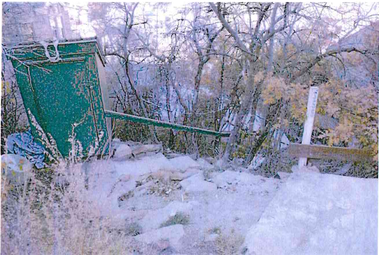
355 Ontario Avenue looking west
