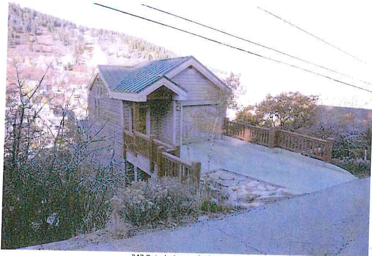
347 Ontario Avenue looking west
