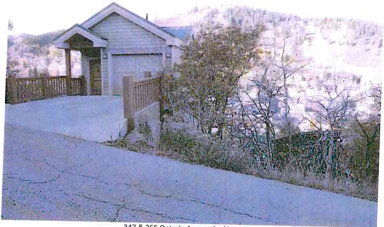
347 & 355 Ontario Avenue looking west
