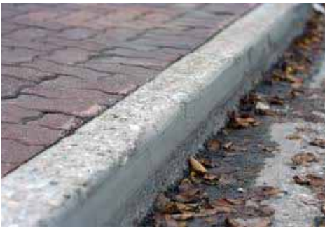
Concrete Curb and Gutter Concrete Paving
