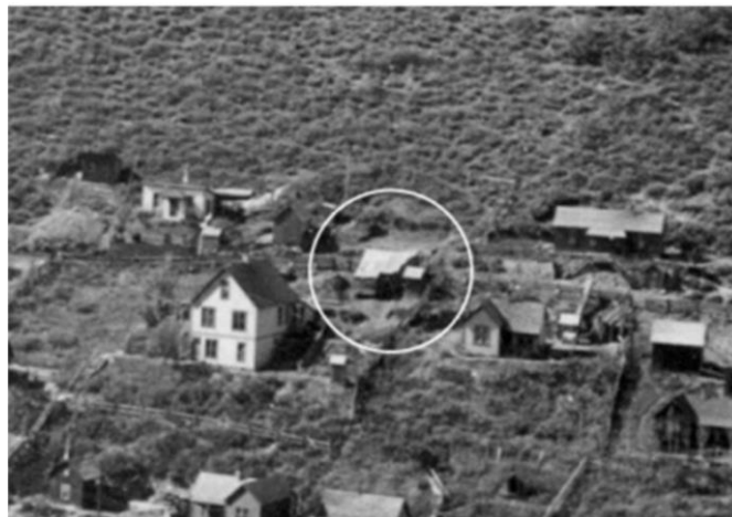
C. 1904 photograph showing the shed roof sloping away from Utah Avenue.
