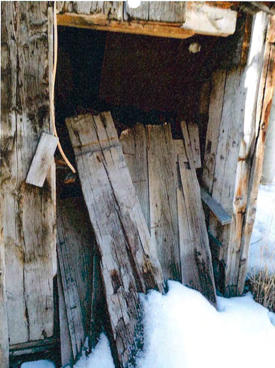
addition to garage
