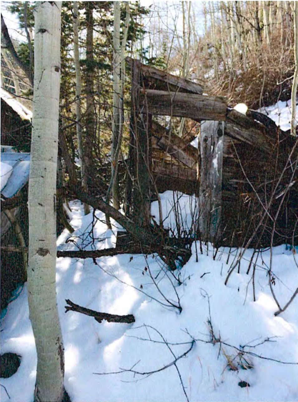
Small shed to rear of accessory structure/garage
