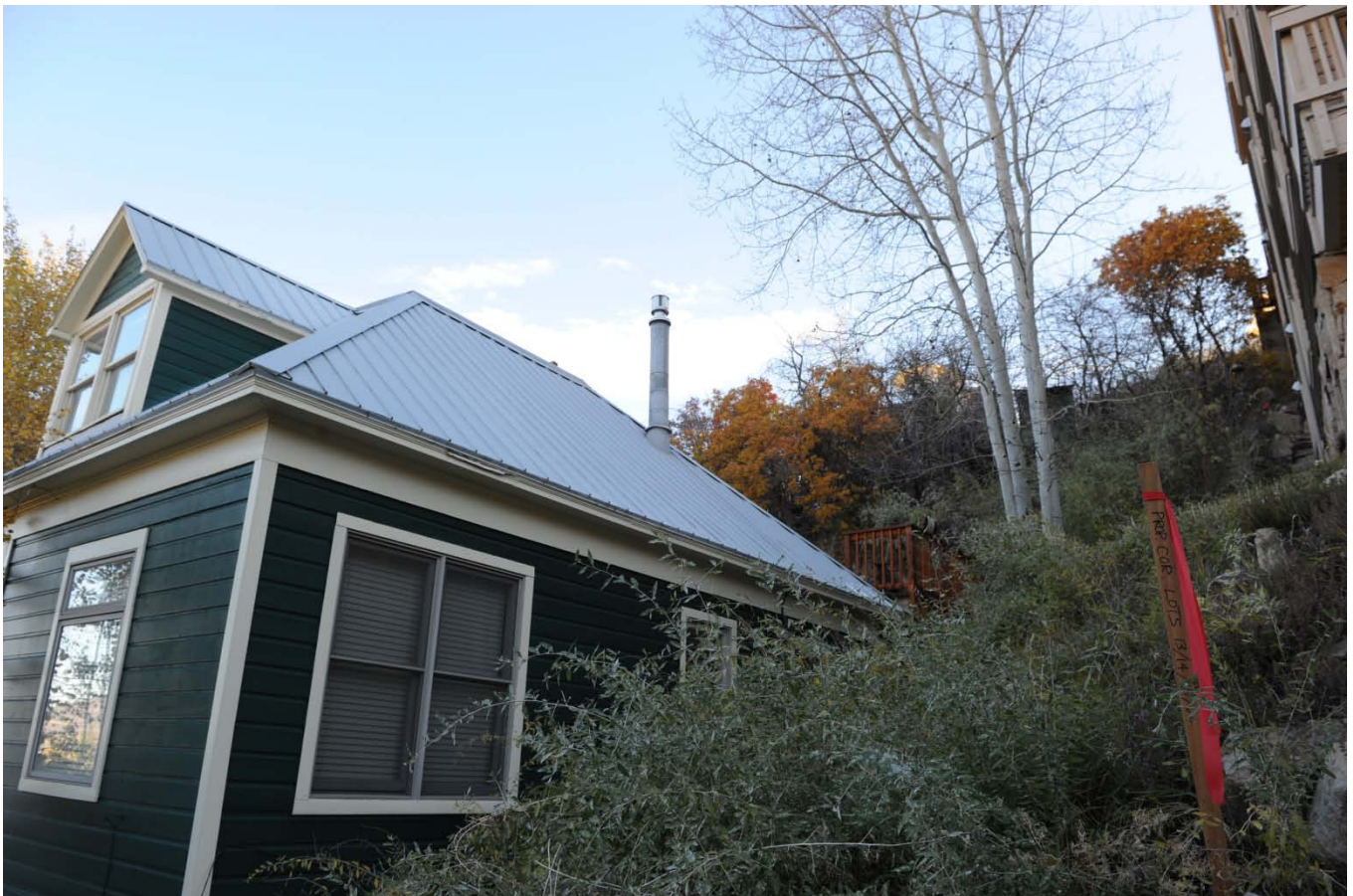
355 Ontario Avenue looking east
