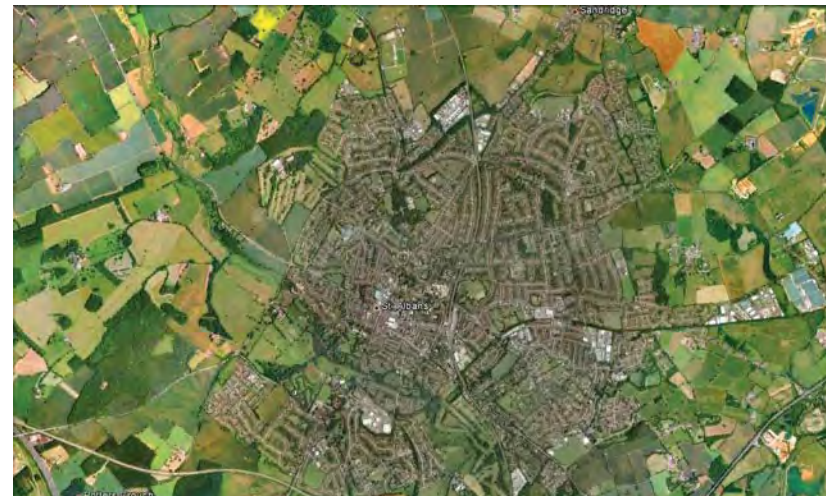
View of St. Albans, UK from Google Earth. Development continues to evolve within the urban center promoting urban reinvestment while protecting local agriculture and open space.
