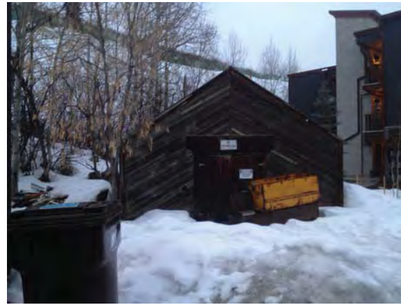
ENTRY WALL/ WEST
