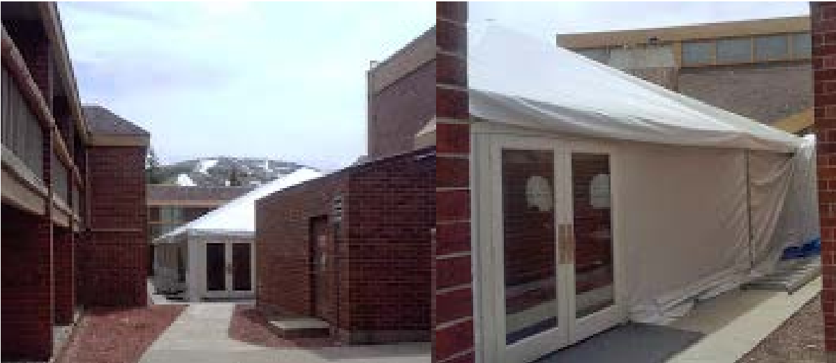
Entrances into the enclosed tent within the Yarrow Hotel Courtyard
