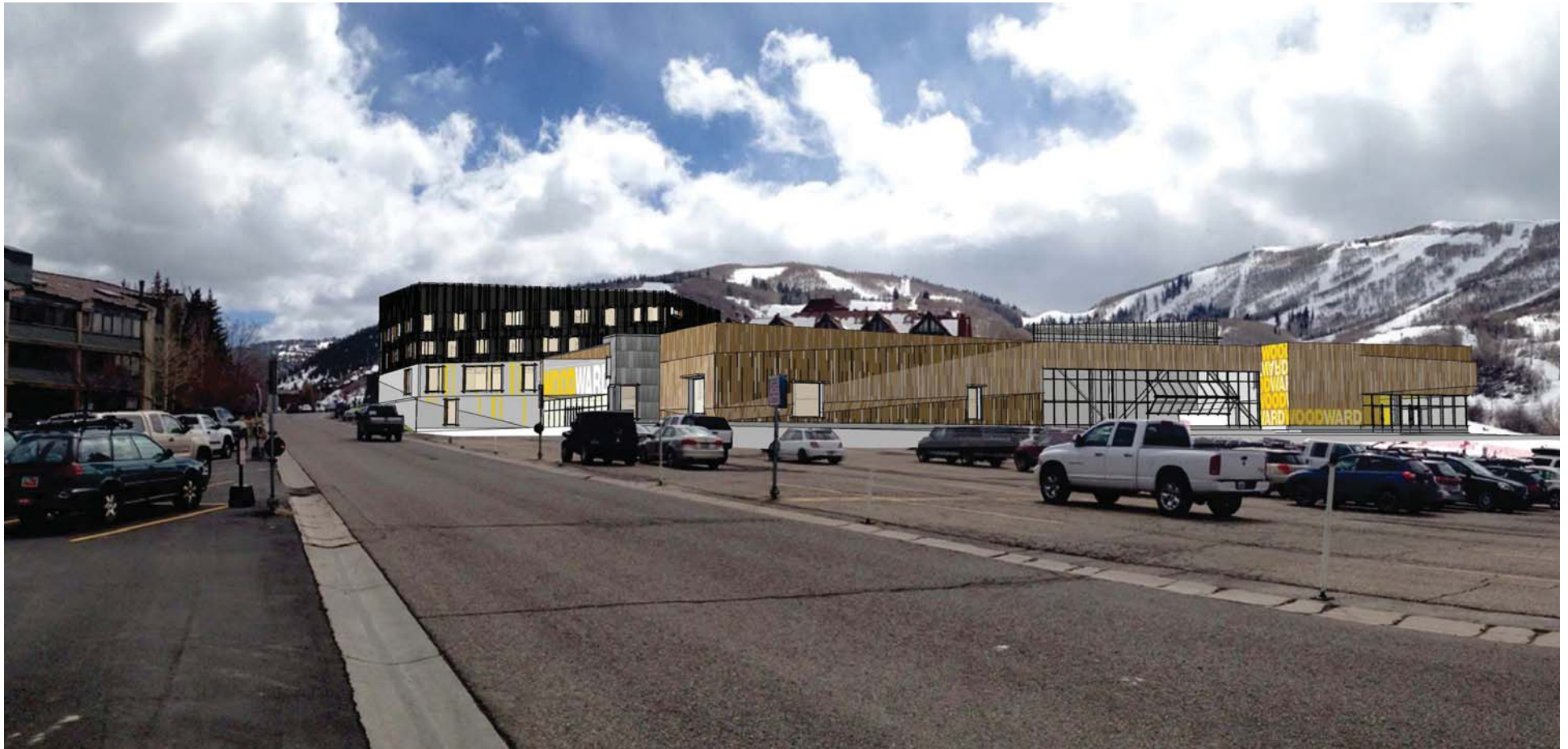
VIEW SOUTH FROM EXISTING SURFACE PARKING ENTRANCE
