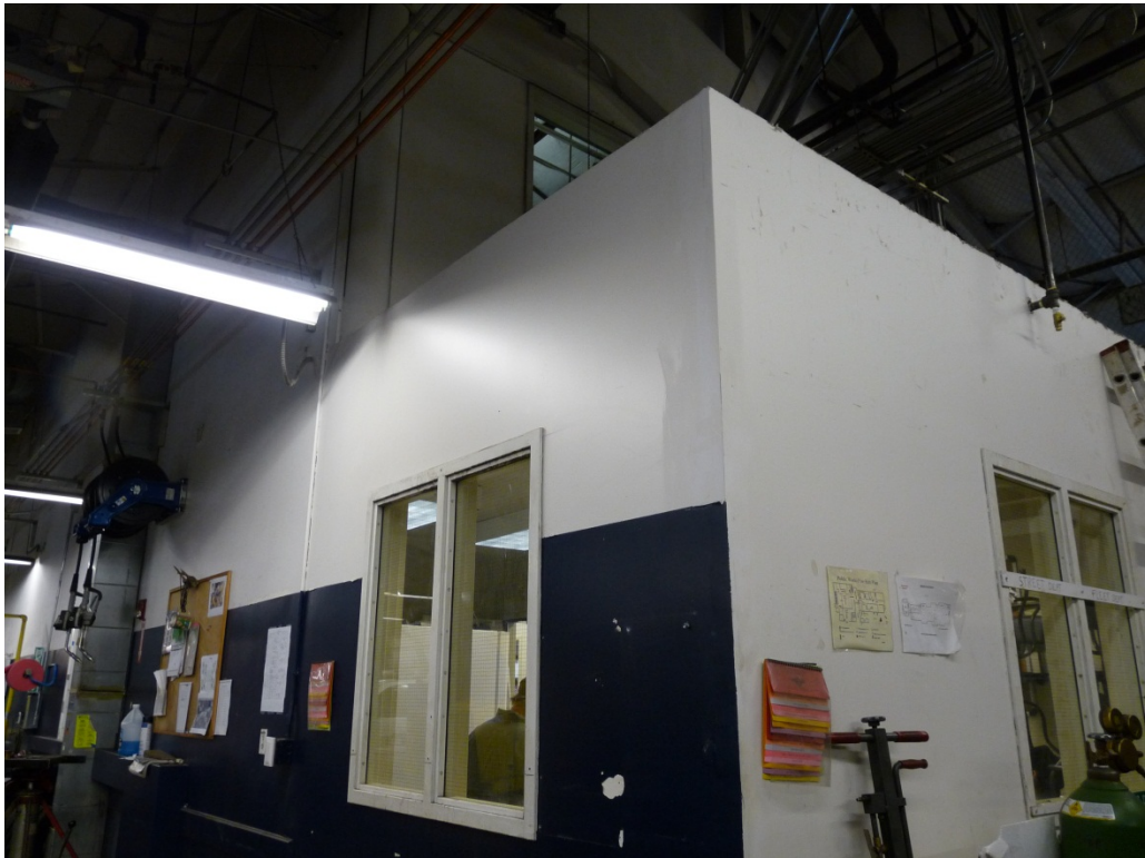
FIGURE B.1-4: EXISTING SPACE ADJACENT TO THE REPAIR AREA
