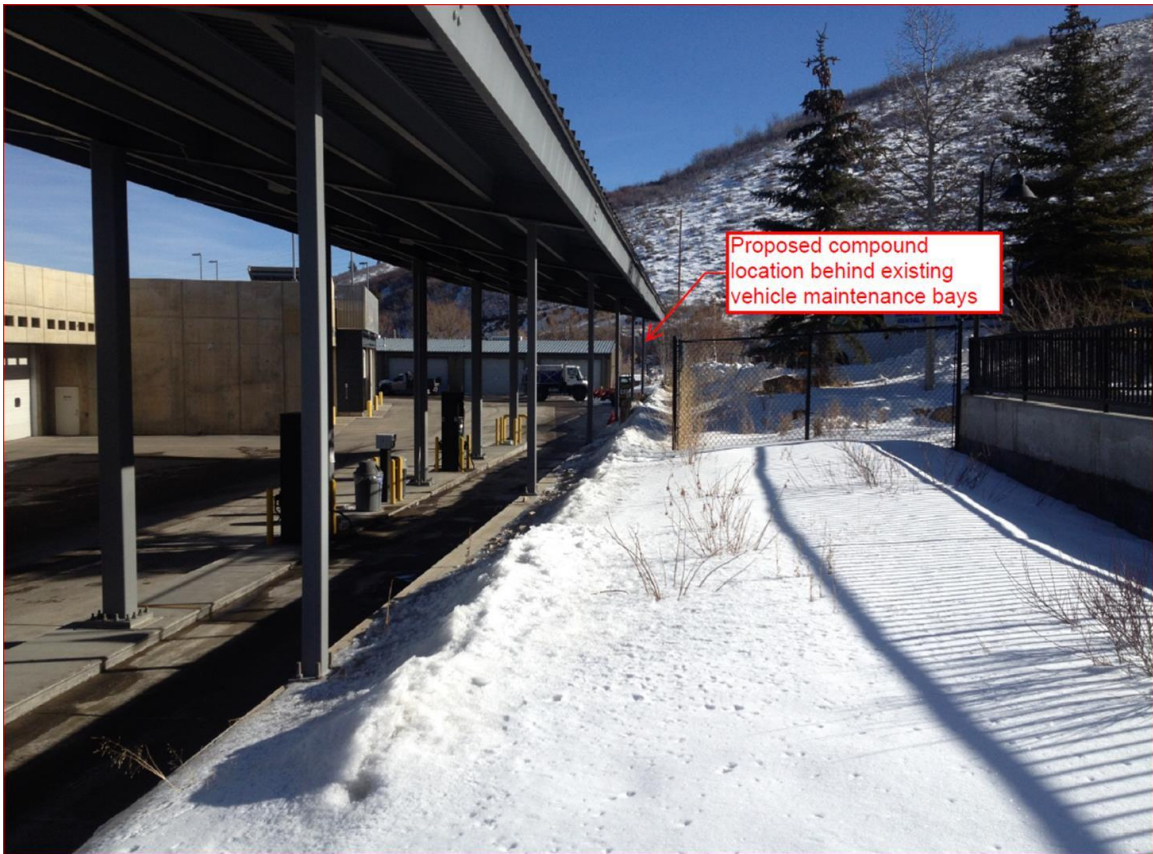
Figure 10. Existing Fueling Canopy and Proposed Compound Location
