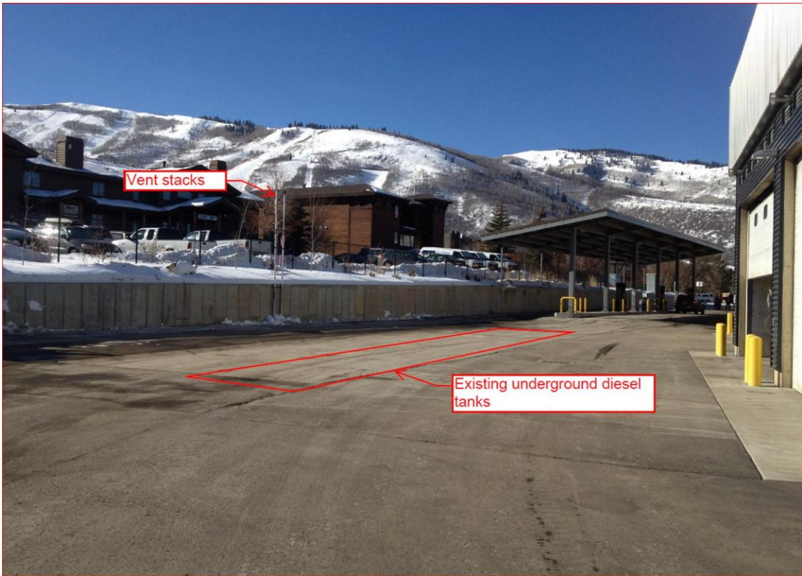
Figure 9. Existing Underground Storage Tanks
