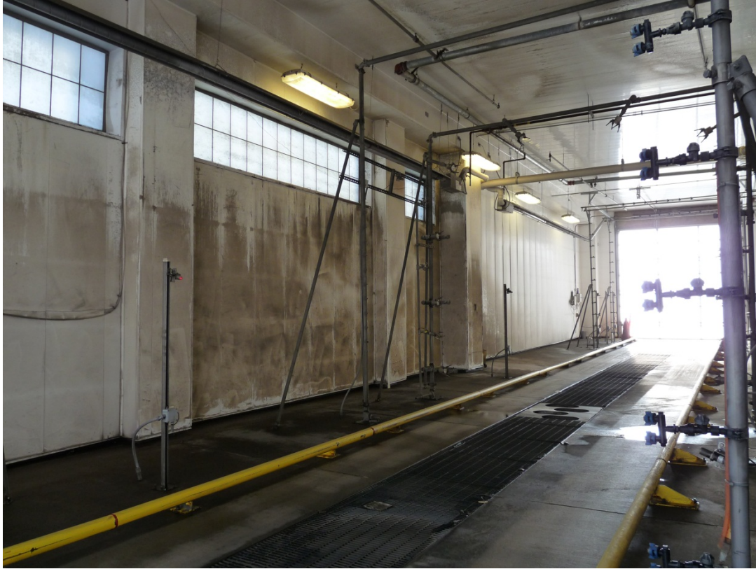
FIGURE B.1-9: EXISITNG WASH BAY
