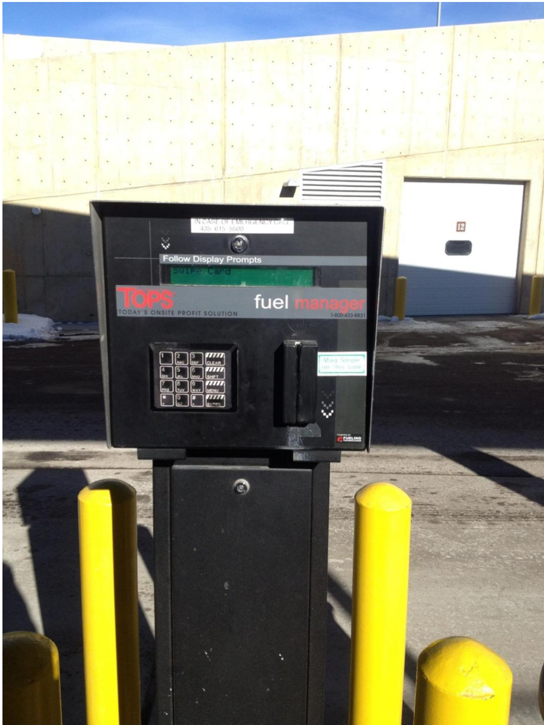
Figure 8. Existing Fuel Management System
