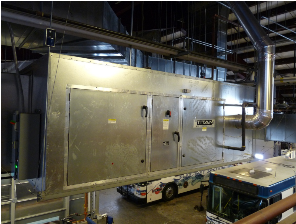
FIGURE B.1-6: EXISTING MAKEUP AIR UNIT
