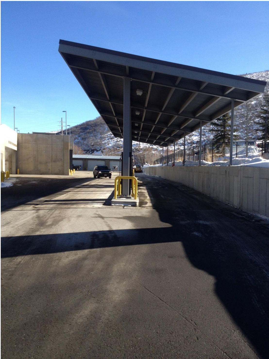
Figure 5. Existing Fuel Island
