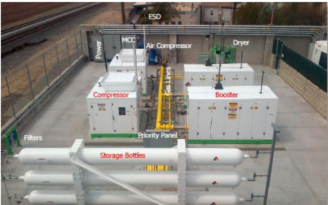
Figure 4. Typical CNG station design and configuration
