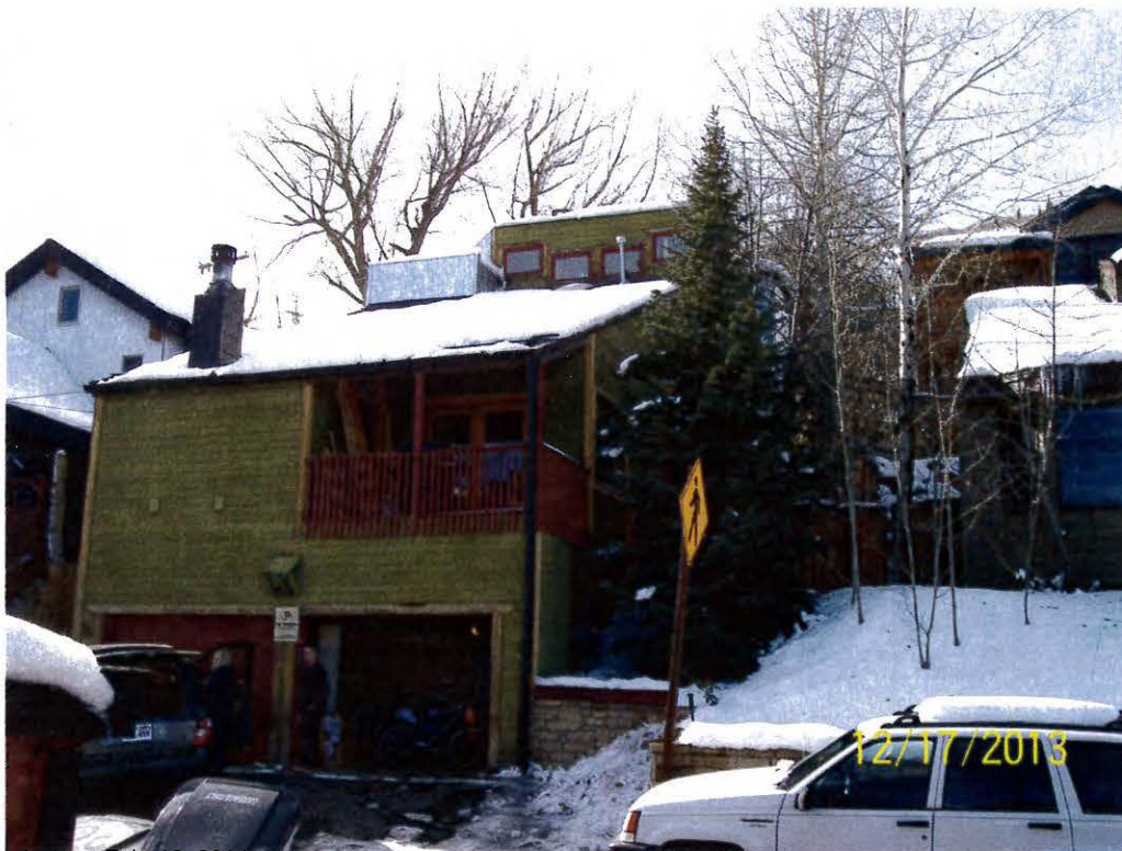
12/17/2013 Adjacent home to the south
