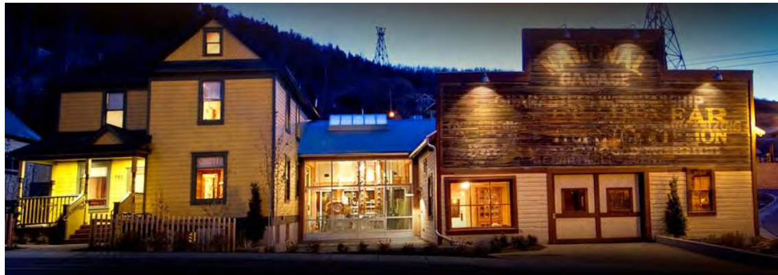
The High West Distillery, shown prior to restoration above and post-restoration below, was a very successful project illustrating the adaptive reuse of two historic buildings - the Beggs House (1914) and the Watts Garage (1907).
