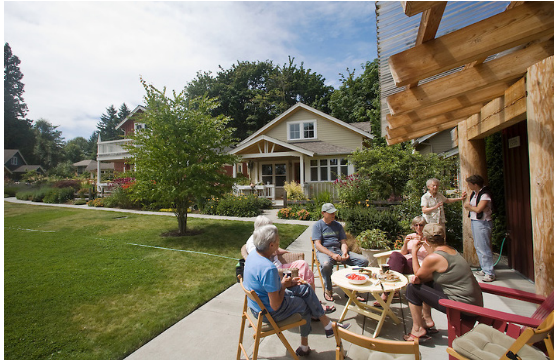
Conover Commons Cottages located in Redmond, WA is a private development made up two-bedroom, two-bath, 1000 square foot homes.
