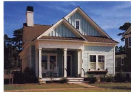
Porch roof forms are consistent with home
