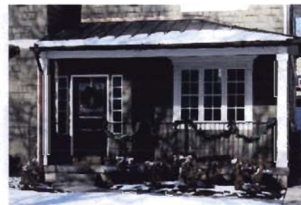
Porches are elevated 18" 8" above finished grade
