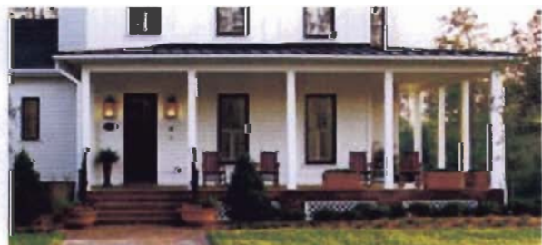
Porch raised a minimum of 18" 8" above finished grade
