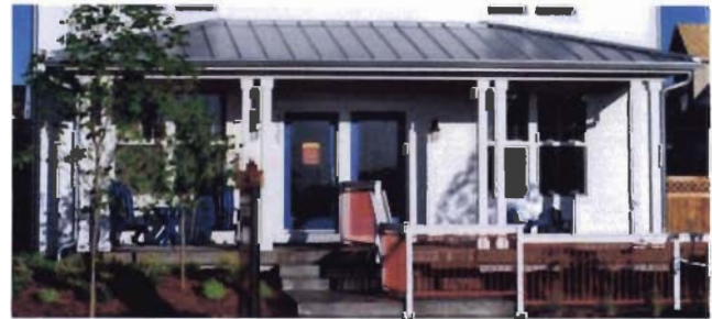
Properly detailed porch elements
