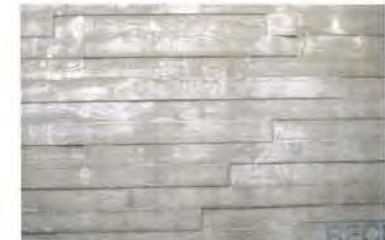
BOARD-FORMED CONCRETE RETAINING WALLS
