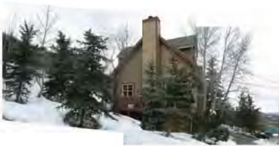
4 SOUTH - INTO SITE
